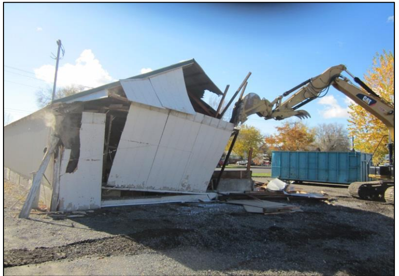
Below: Demolition of Annex Storage Shed
