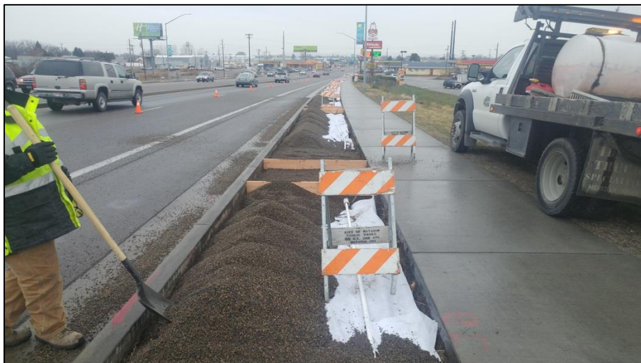
Bottom left: Spreading rock on planter on E. Idaho Ave.
