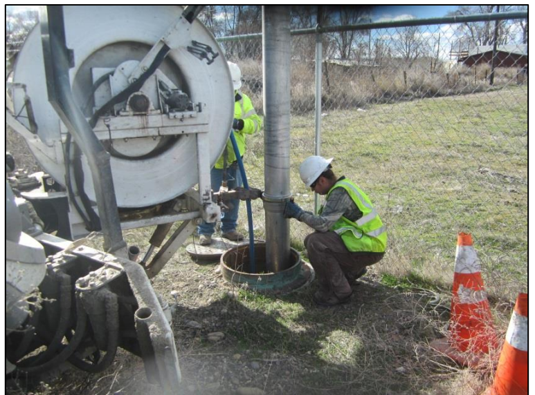
Bottom: Staff cleaning sanitary sewer.
