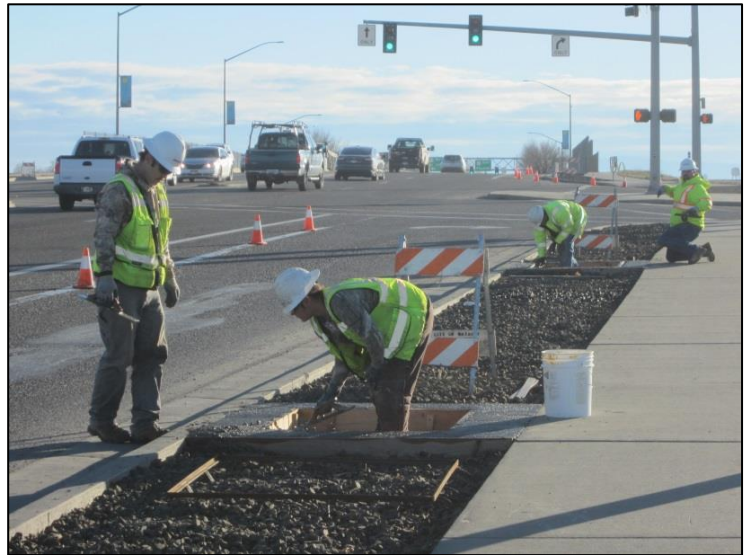
Top: Employees finishing concrete for tree grates on E. Idaho Ave.
