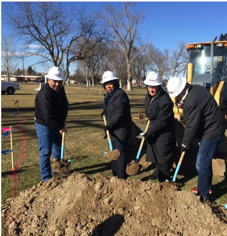
Left: Council members participate in Splash Pad groundbreaking.
