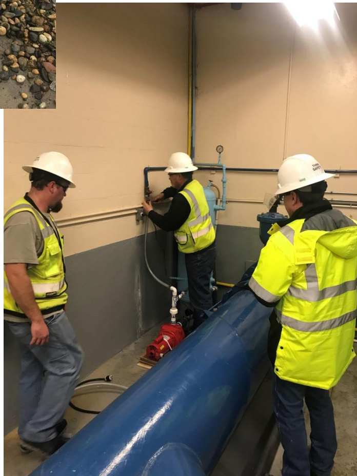
Employees replacing a defective sample pump at Water Treatment Plant.
