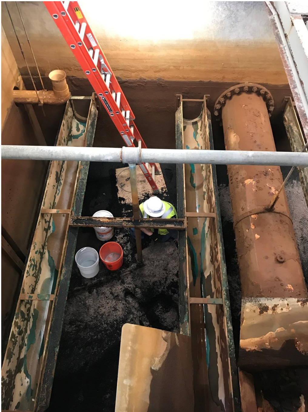
Employee making repairs to filter #2 at old Water Treatment Plant.
