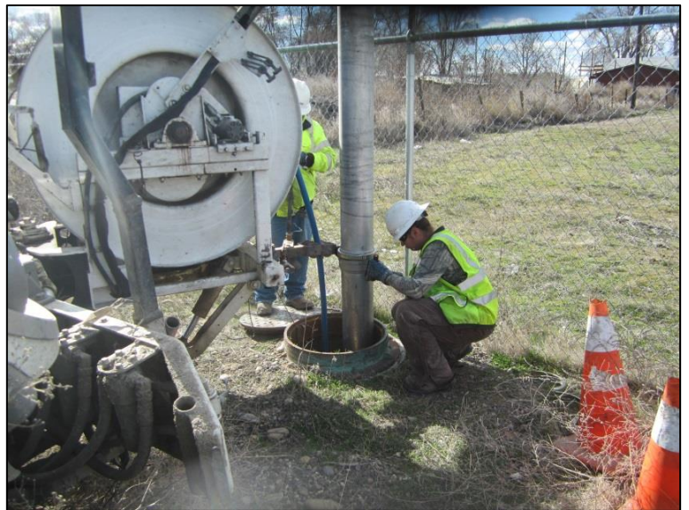
Bottom: Staff cleaning sanitary sewer.
