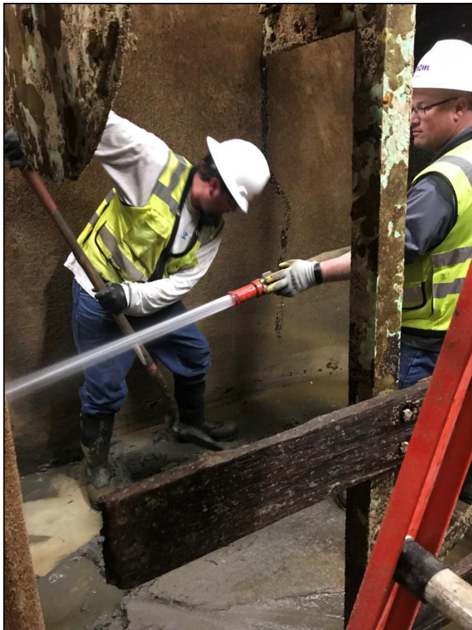
CH2M employees removing sand from Clarifier #1 at Water Treatment Plant.
