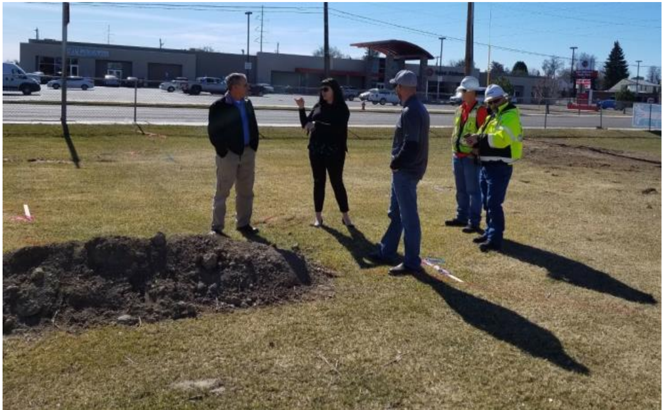
City Staff meeting with CH2M Splash Pad Project Manager and Splash Pad Contractor on site.
