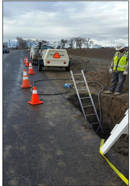
Top: CH2M crew installing water service on SE 2 nd St.
