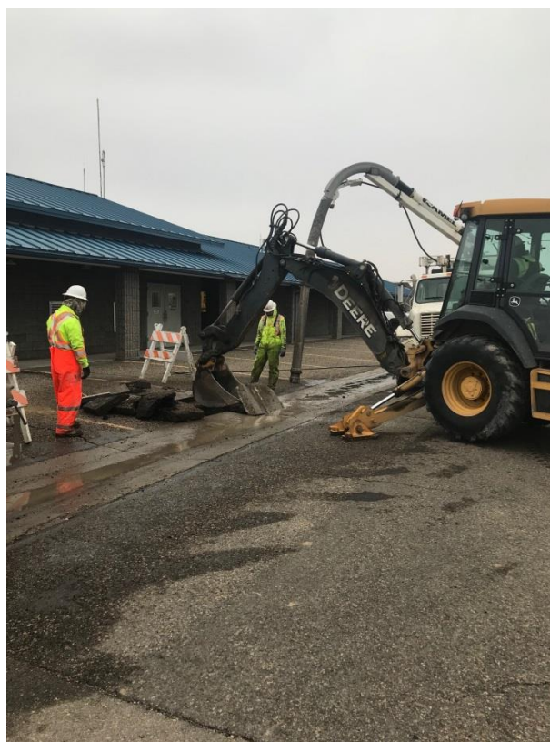
Left : Bill DuChene and Bobby Green installing new aerator on Waste Water Treatment Plant Lagoon #1.
