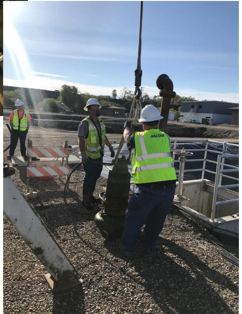
Right: Employees installing backwash water recovery pump #3.
