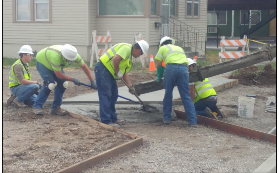
Top: Crew pouring concrete at Annex parking lot.
