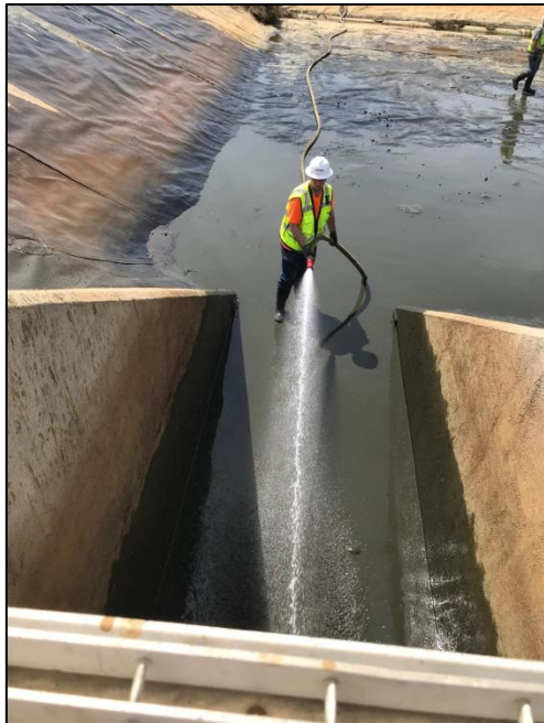
Both: WTP employees cleaning backwash water recovery bed #4.
