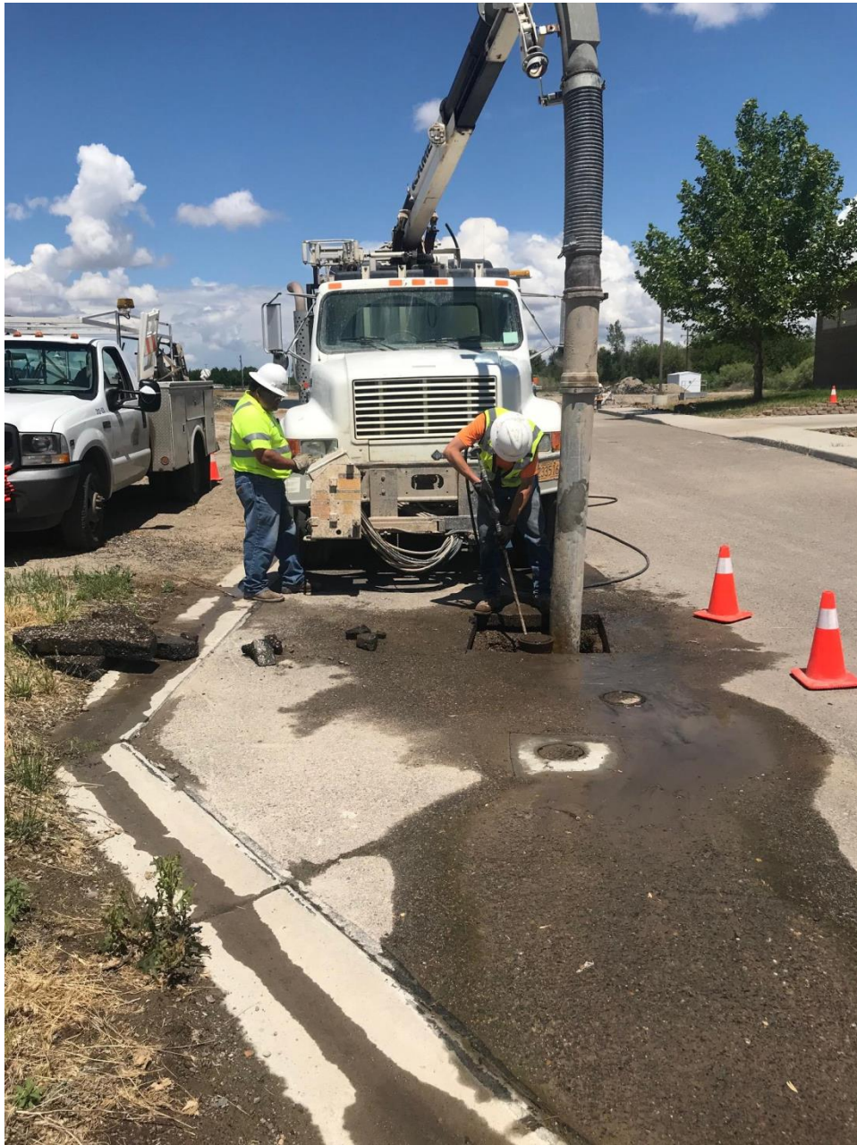
Jacobs employees hydro-excavating leak on well feed line.
