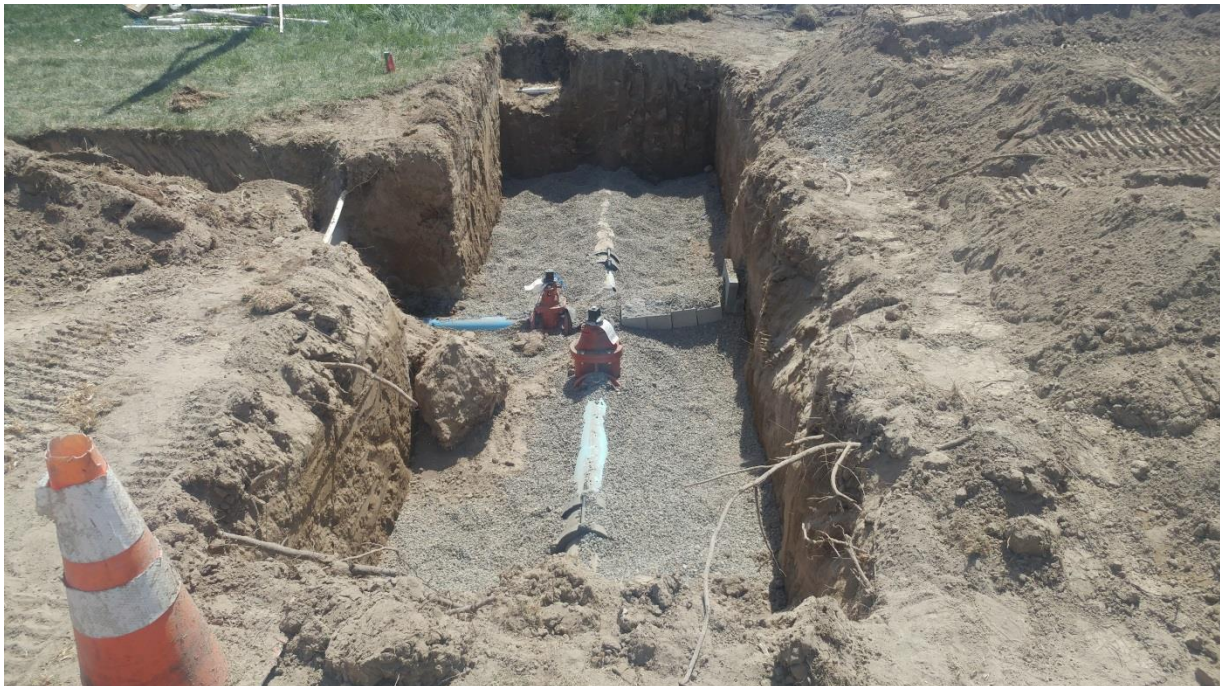
Pipe Modifications at Splash Pad site.
