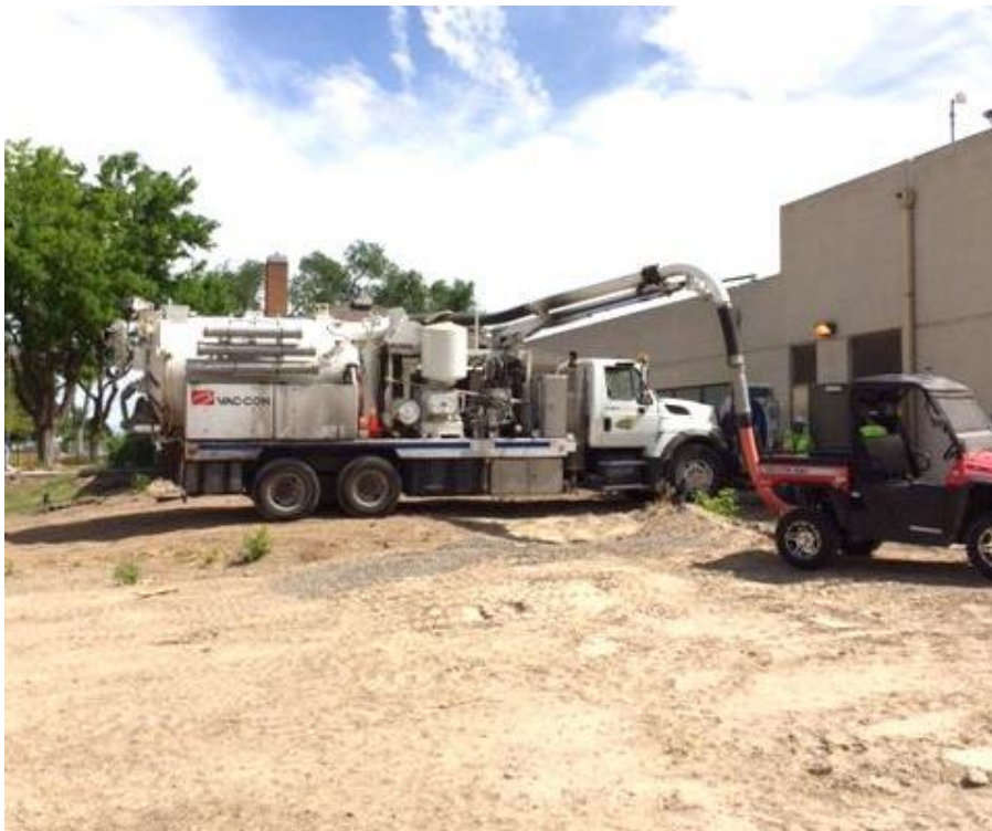
Left: Jacobs crew removing sand media from the old pool building.
