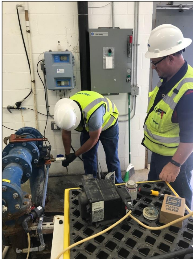
Jacobs employees repairing and modifying the Chlorine injection line at Bench Reservoir.
