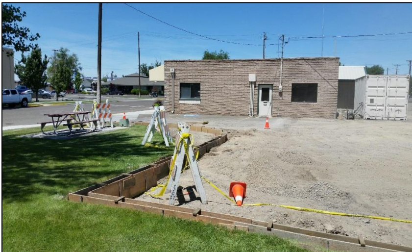
Annex parking lot curb forms.
