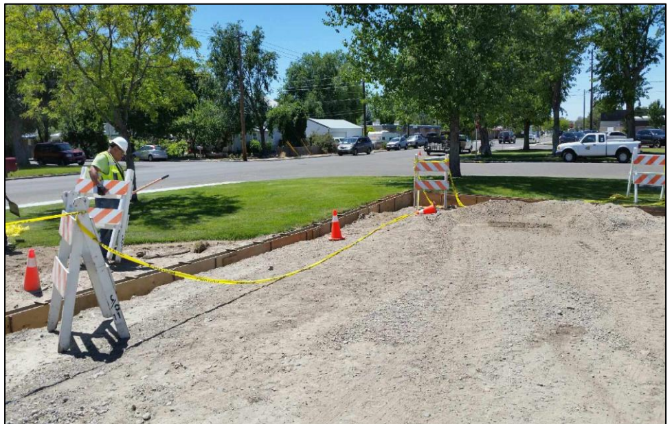
Bottom: Jacobs crew prepping Annex parking lot for paving and curbing.
