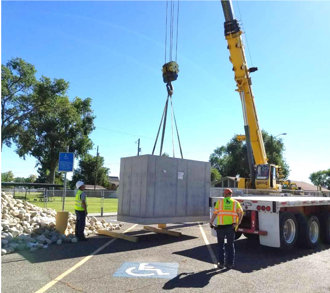
Road Runner Towing off- loading surge tank at Aquatic Center.
