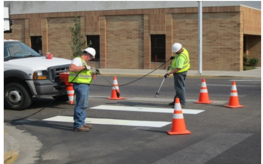
Hot Taping Crosswalks
