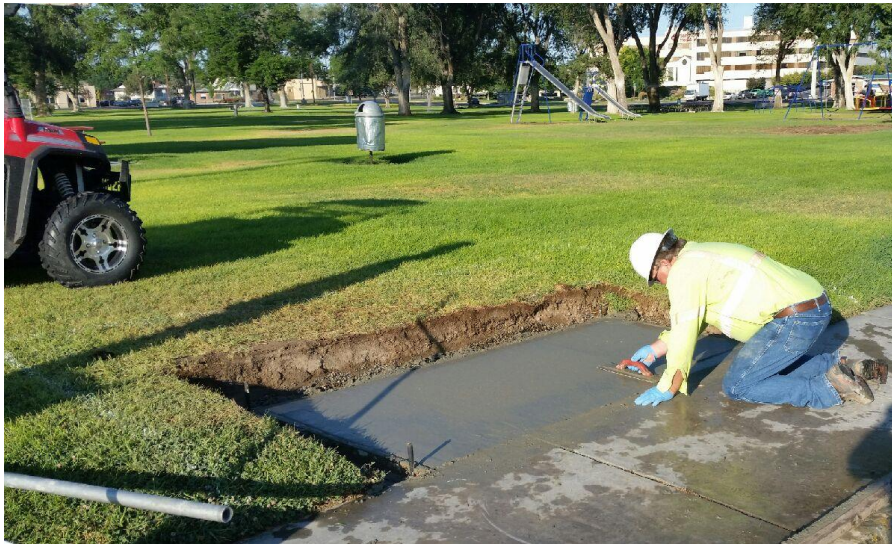
Top: Jacobs employee working on new cement pad for Buddy bench at Lion's Park.
