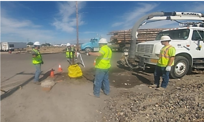
Fire hydrant repair
