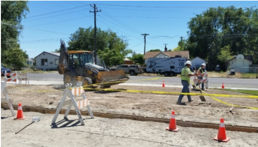
Annex Parking Lot Construction
