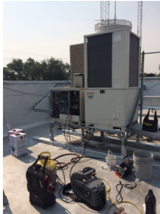
Maintenance on HVAC system
