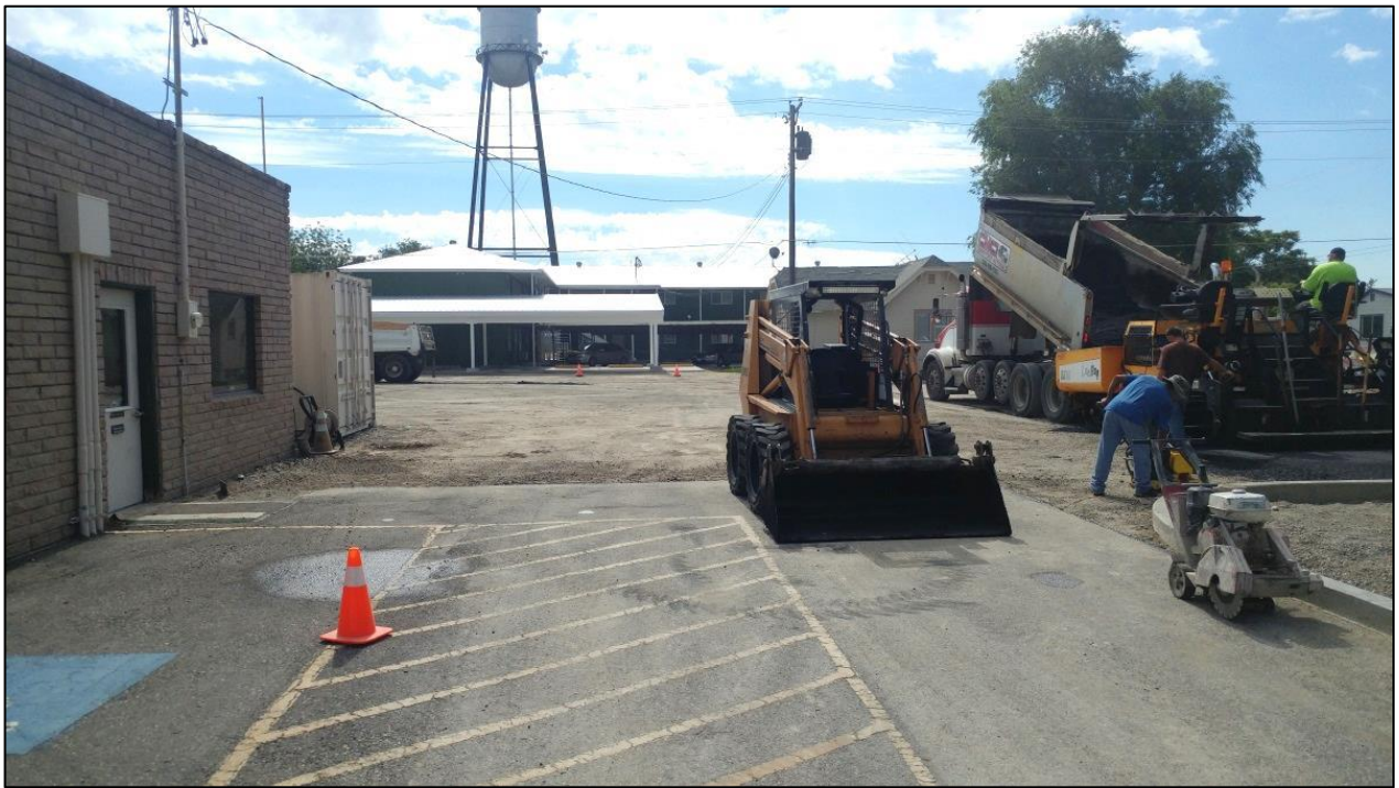
SunRoc paving parking lot at Annex building.
