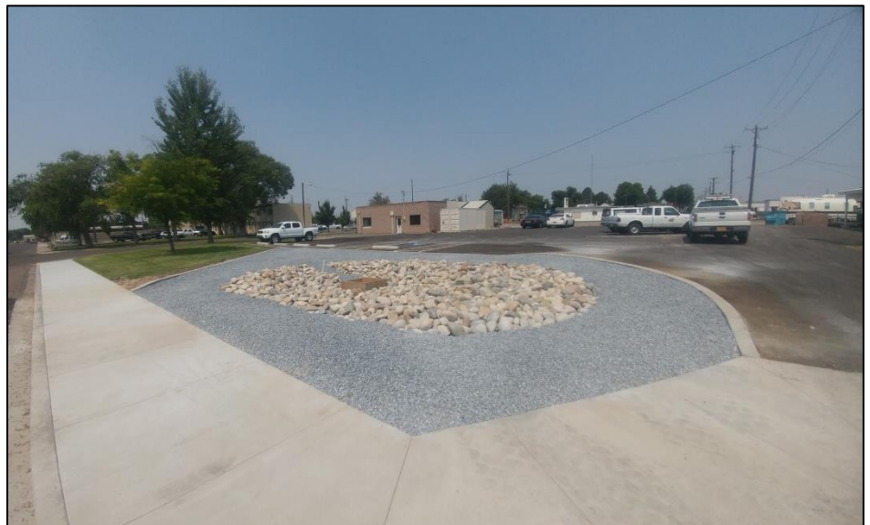
Bottom: Completed drainage swale for Annex parking lot.
