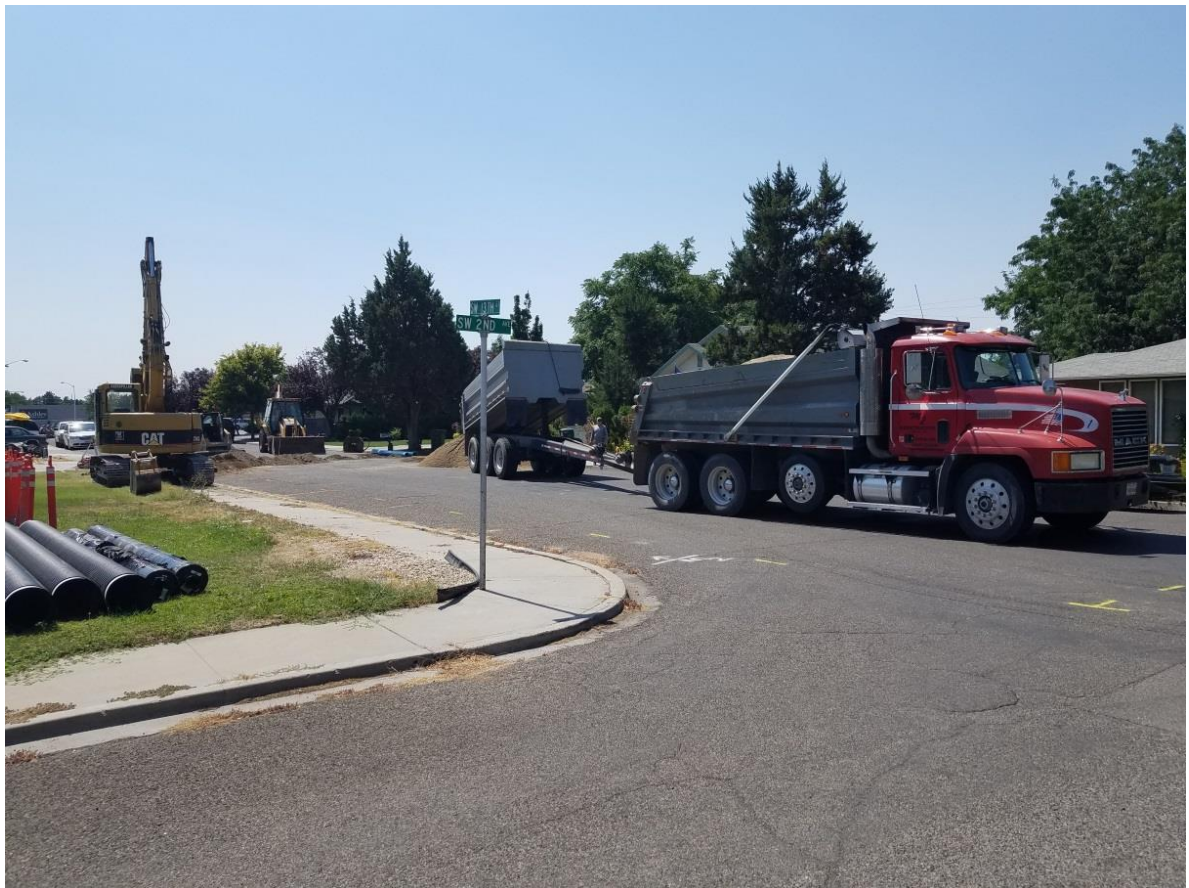
Contractor performing Storm Water Project work.
