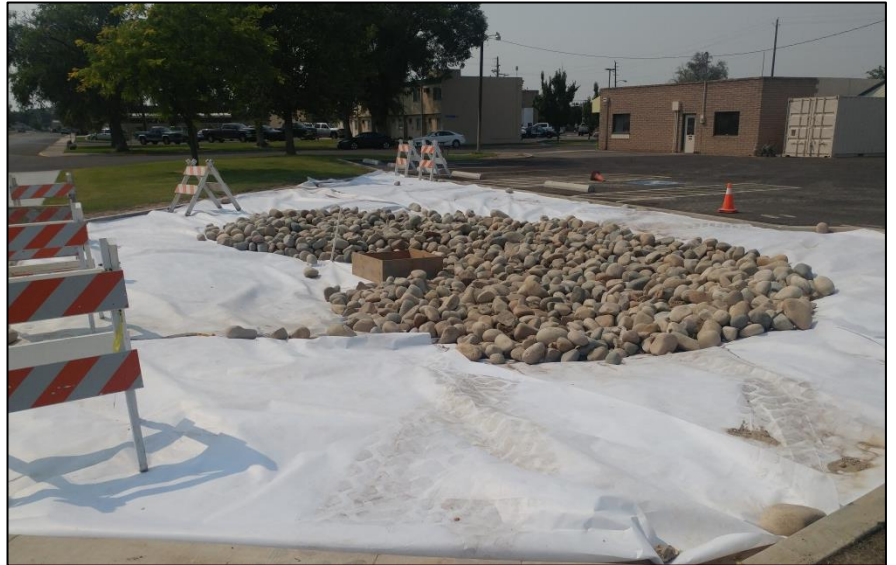
Top: Unfinished drainage swale for Annex parking lot.
