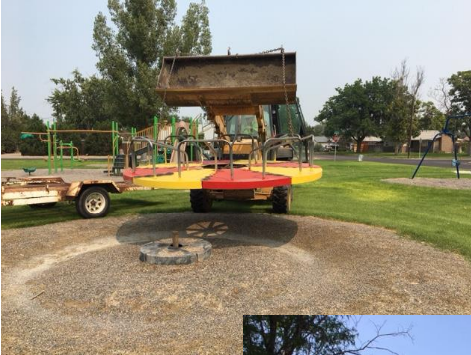
Jacobs crew removing Merri-Go-Round from Laxon Park for repairs.
