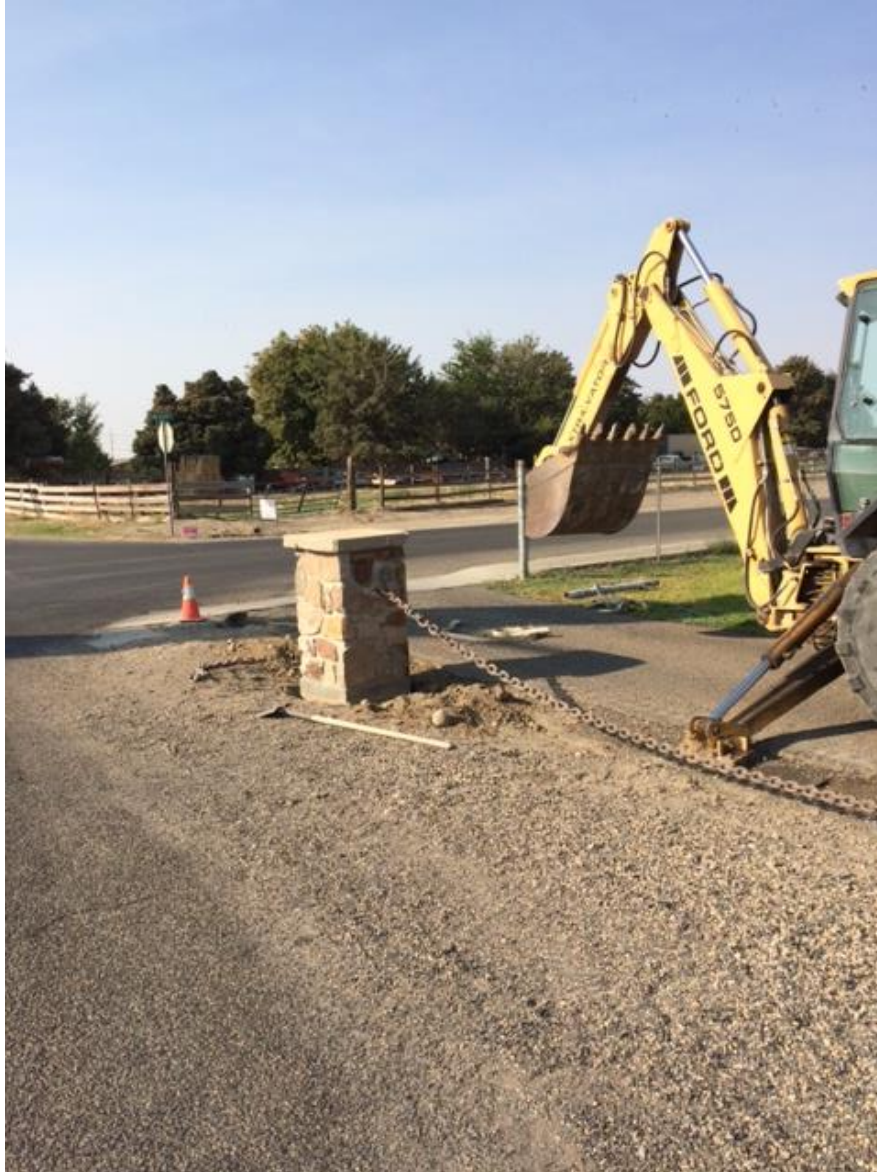
Repairing pillar at Evergreen Cemetery.
