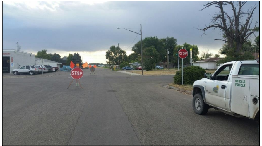
Top: New stop signs installed at SE 3 rd Ave./SE 3 rd St.
