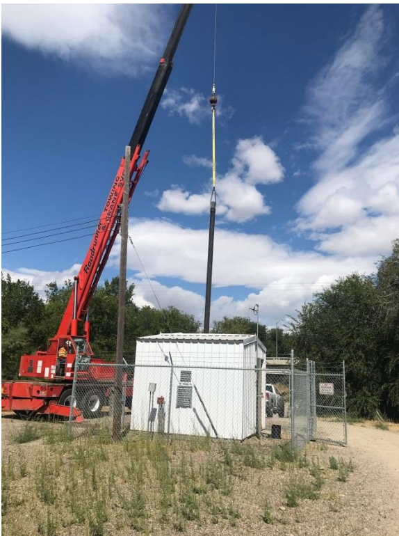
Left: Installation of new pump and column on Well #4.
