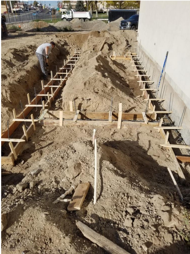
Right: Warrington Construction pipe bursting water main on SW 3 rd Ave.
