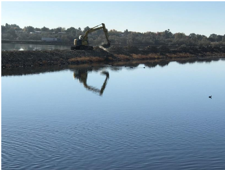
Both: Contractor rebuilding lagoon dikes that were damaged during winter ice storms.
