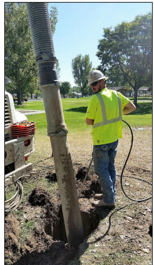
Bottom: Jacobs crew excavating for leak at Lion's Park.
