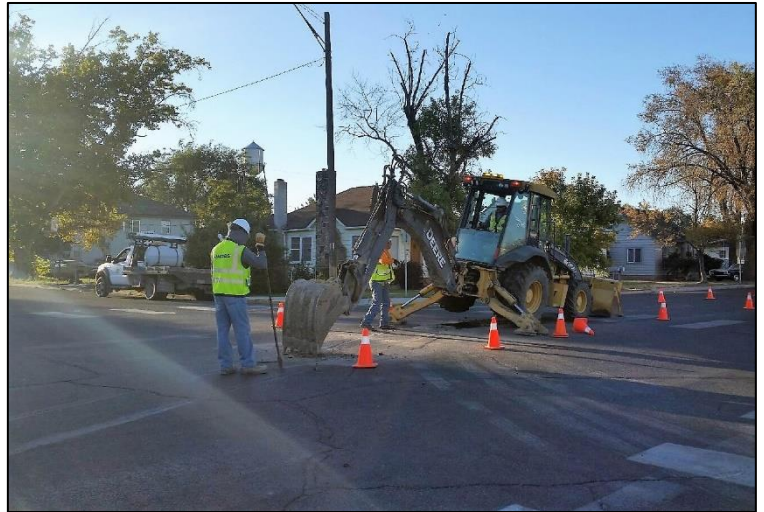
Top: Crew repairing sink hole in asphalt.
