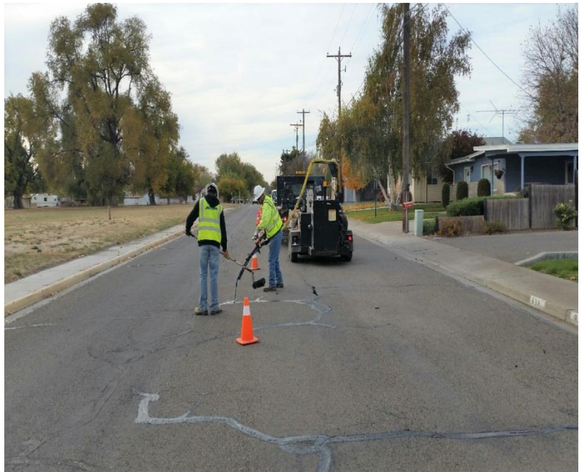
Crew crack sealing in Northwest area of town.
