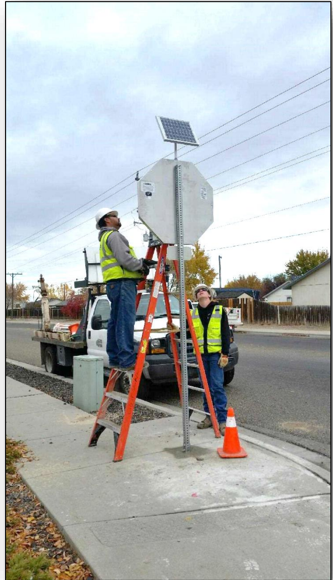
Crew installing new LED Stop sign at intersection of NW 4 th Ave. and Verde Dr.
