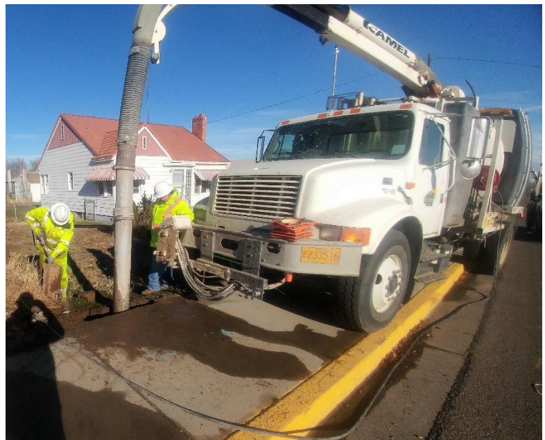
Crew installing new water service on SW 4 th Ave.
