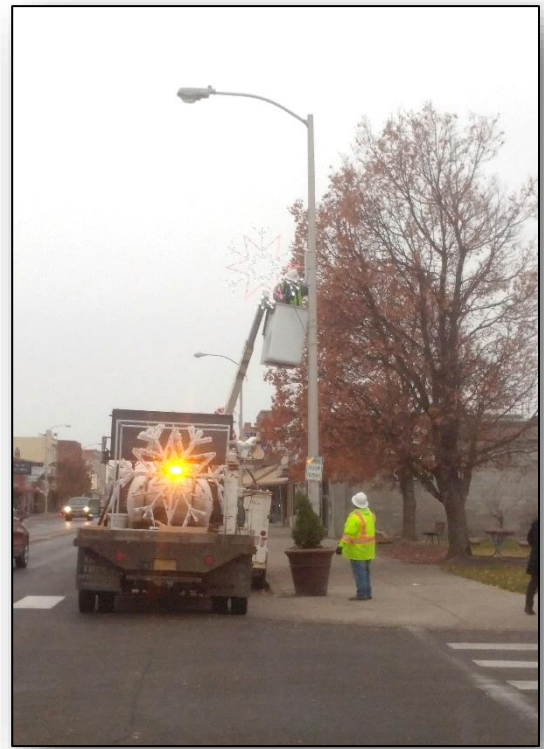
Top: Crew installing new Holiday ornaments on S. Oregon St.
