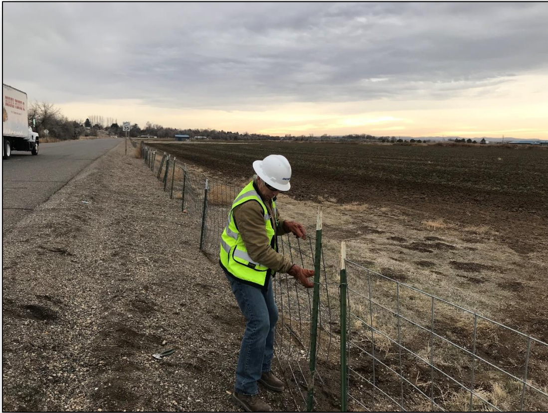
Treatment employee repairing perimeter fence at WWTP.
