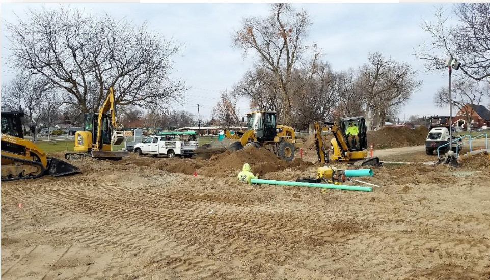
Both: Splash Pad site construction
