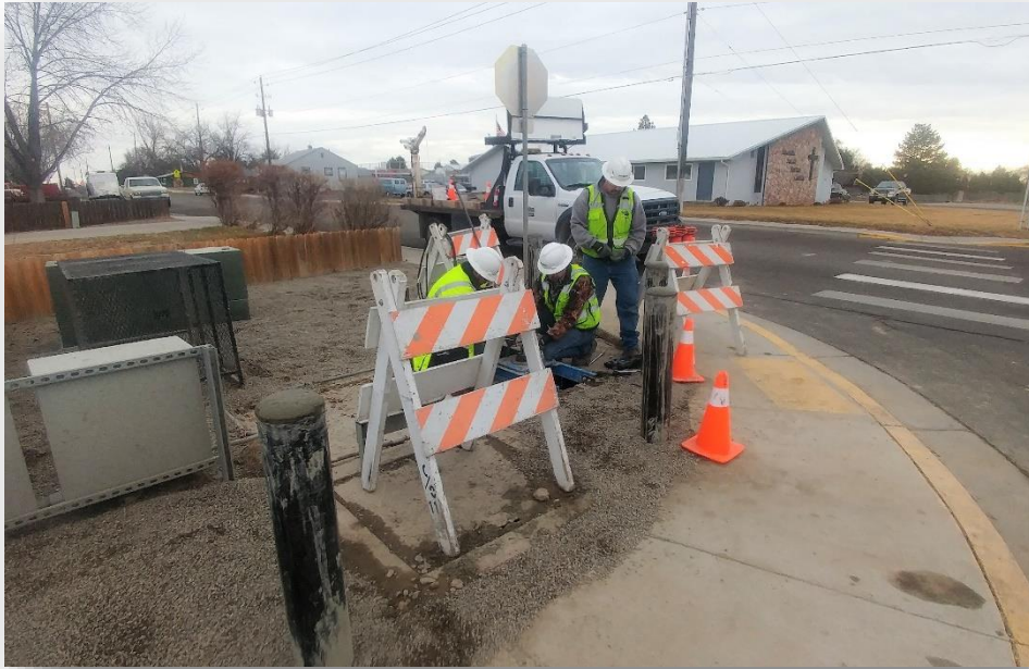
Top: Crew installing bollards and working on Verde Irrigation Pump.
