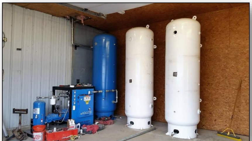
Bottom: New compressor and air tanks.
