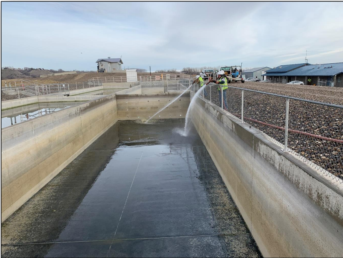
Staff cleaning contact chamber at WWTP.
