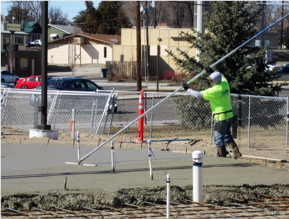
Both: Contractors finishing Splash Pad concrete.
