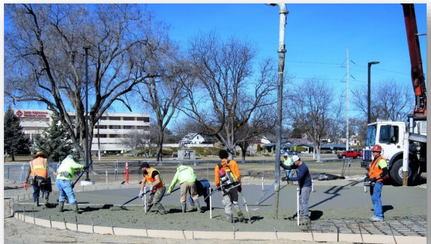
Both: Contractors pouring Splash Pad concrete.
