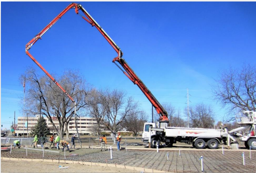
Both: Contractors pouring Splash Pad concrete.
