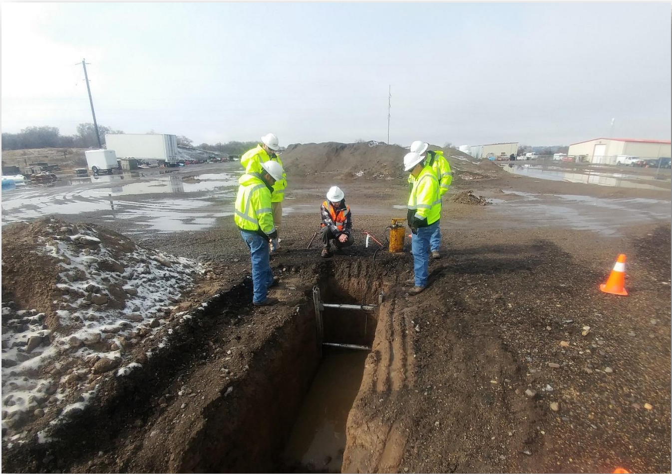
Staff completing Excavation Competent Person Training.
