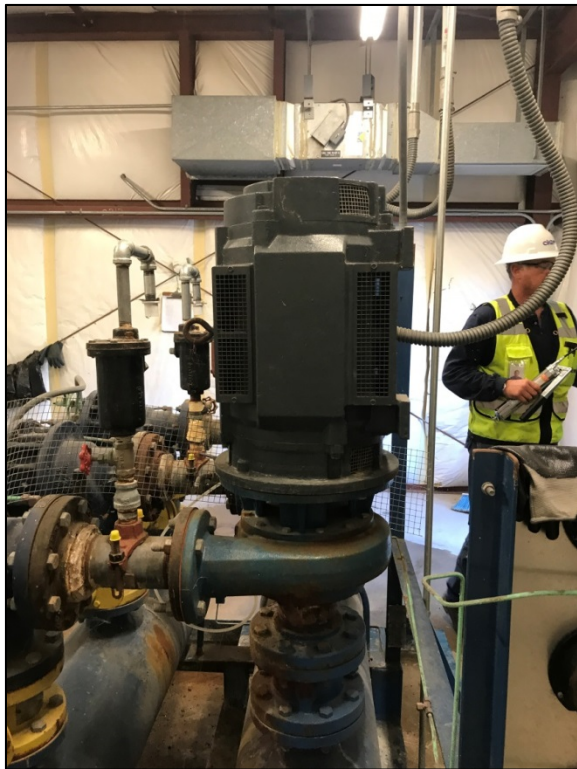
Water Treatment Plant employees lubricating pump bearings.
