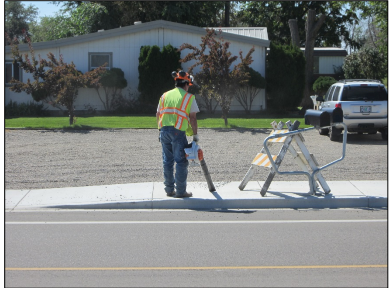
Field Services crew blowing chips off sidewalks.
