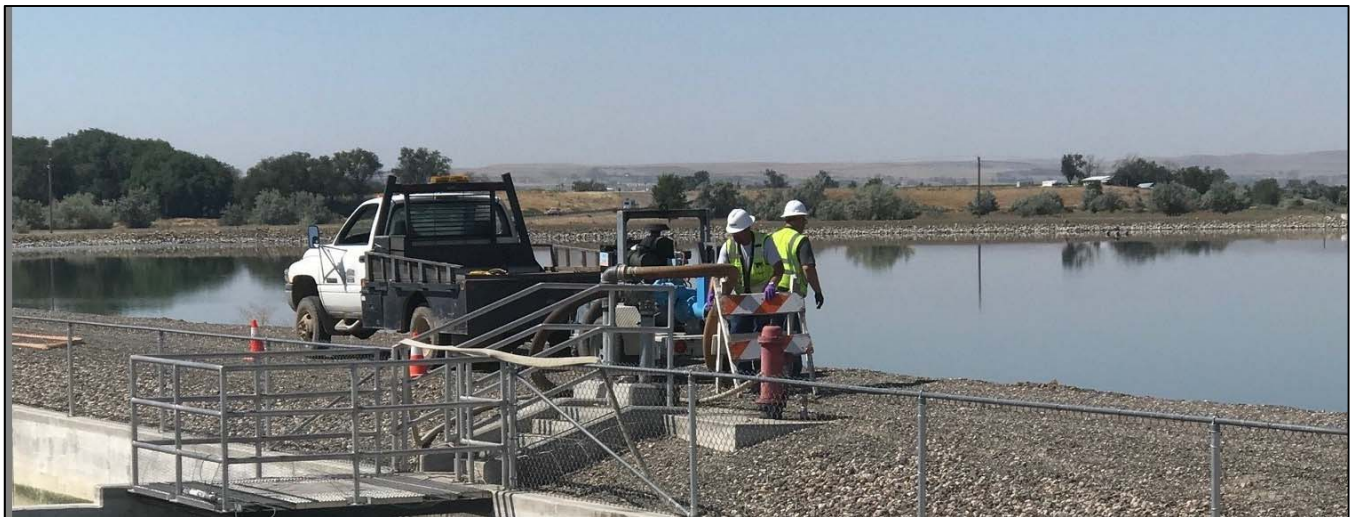
Chlorine contact basin No. 2.
