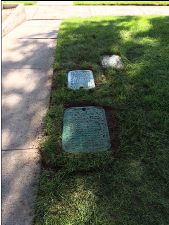
Water valves installed at Ontario City Hall in the lawn next to the South employee parking lot and Ontario Apartments.
