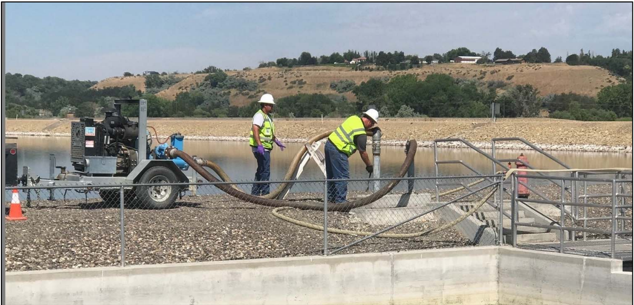
Cleaning chlorine contact basin No. 1 at WWTP.
