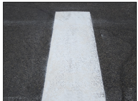
Field Services crew hot taping crosswalk bars.
