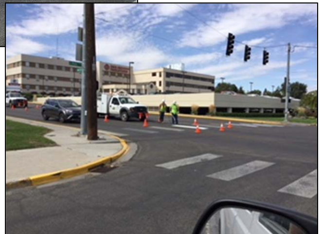
Field Services Crew installing hot tape crosswalk bars along North Oregon Street (above) and SW 4 th Avenue (right).
