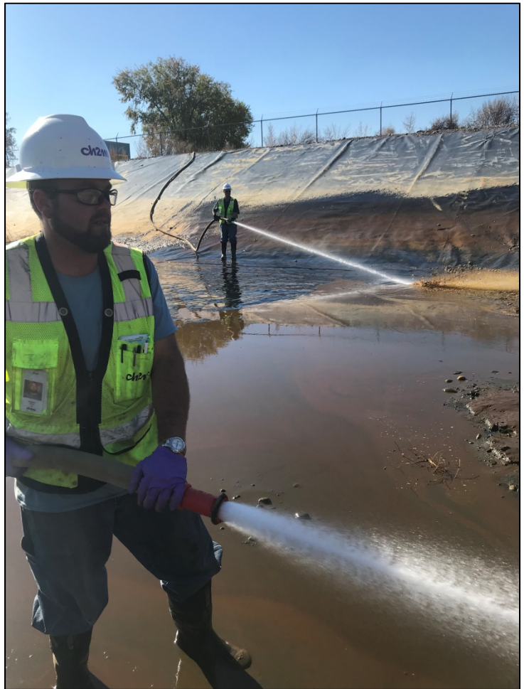
Employees cleaning one of the settling ponds at Water Treatment Plant.
