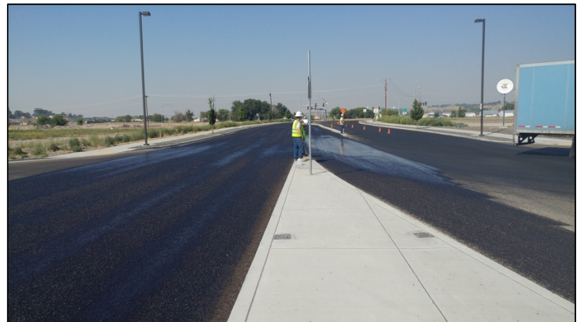
Traffic control along NW Washington Avenue during fog coat after chip seal.
