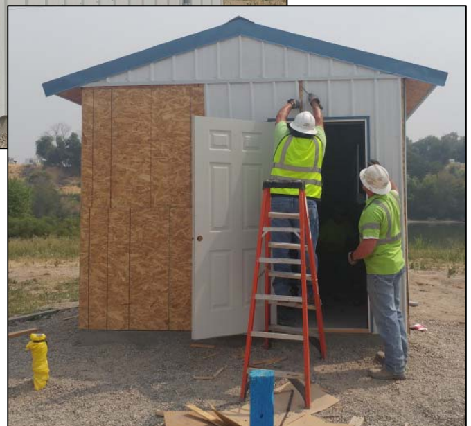
Field Services crew finishing the well house for Well No. 17 at the Water Treatment Plant.
