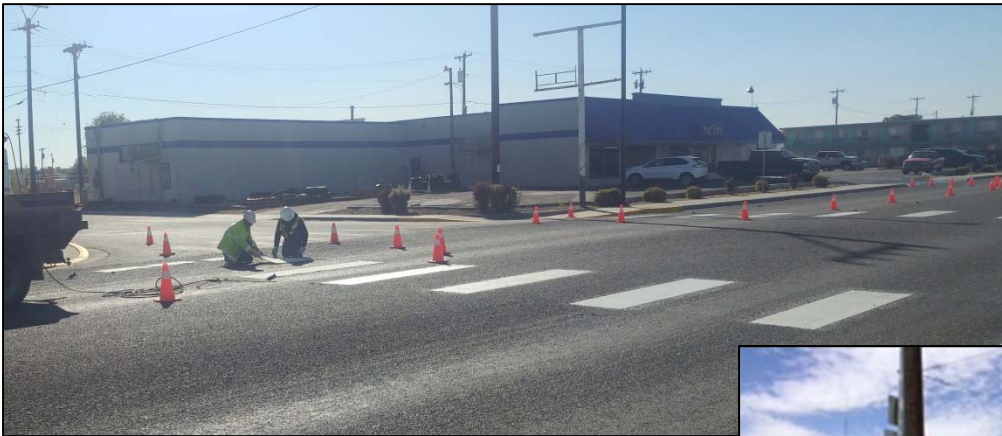
Field Services Crew installing hot tape crosswalk bars along North Oregon Street (above) and SW 4 th Avenue (right).
