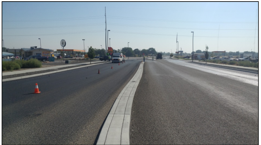
Moving traffic along NW Washington Avenue during application of fog coat.
