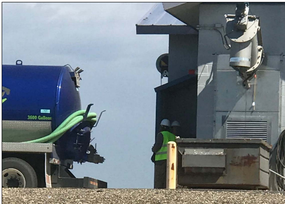
Septage Receiving Plant receiving a load.
