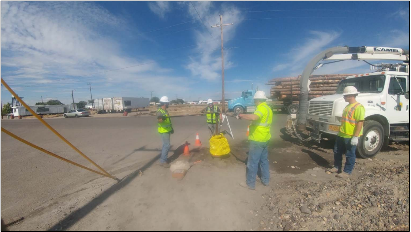
Removing foot-valve out of Fire Hydrant on NE 3 rd Ave.
