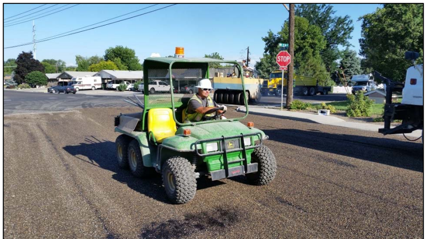
Field Services Crew chip sealing NW 2 nd Avenue and NW 4 th Avenue.
