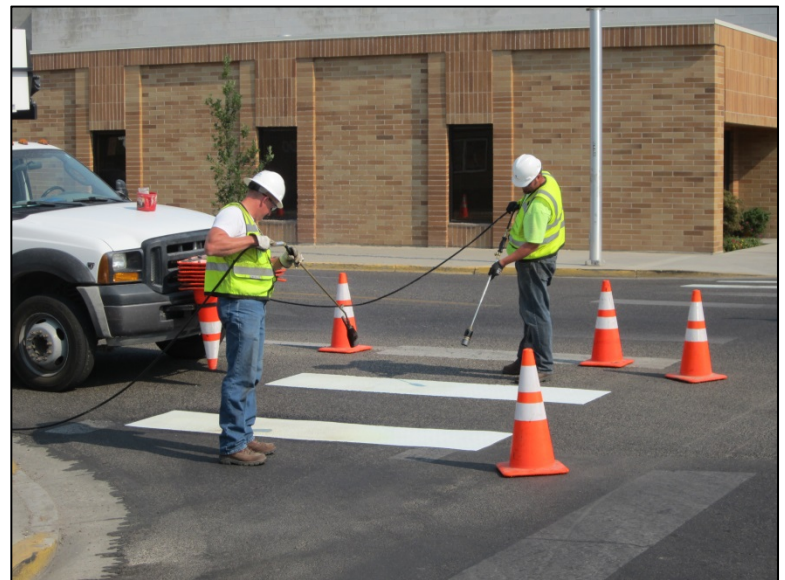
Field Services crew hot taping crosswalk bars.
