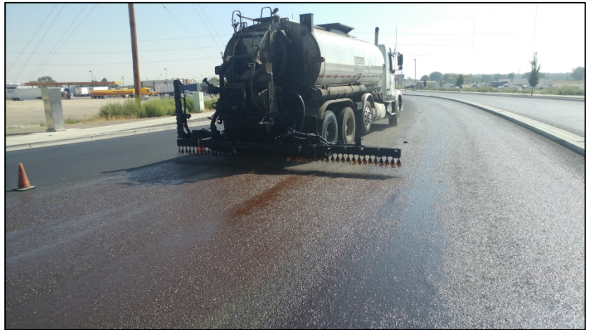
Field Services Crew applying fog coat on NW Washington Avenue.
