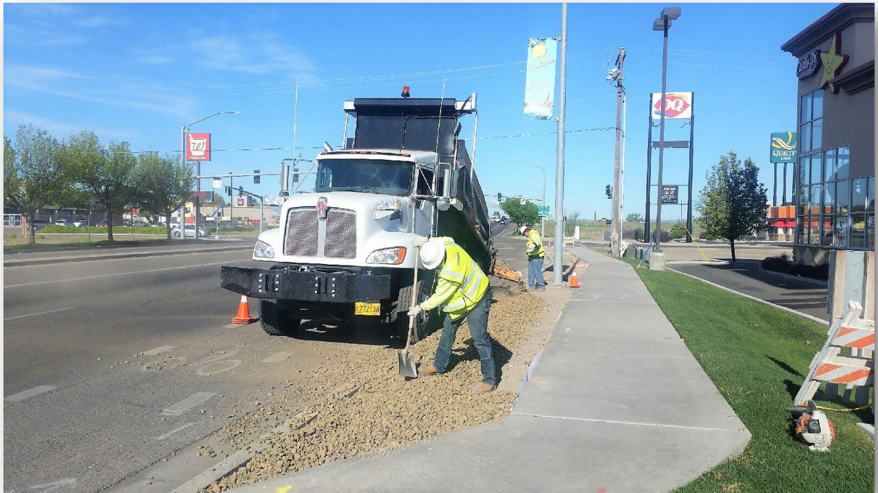
Jacobs crew installing new rock in planter strip on E. Idaho Ave.
