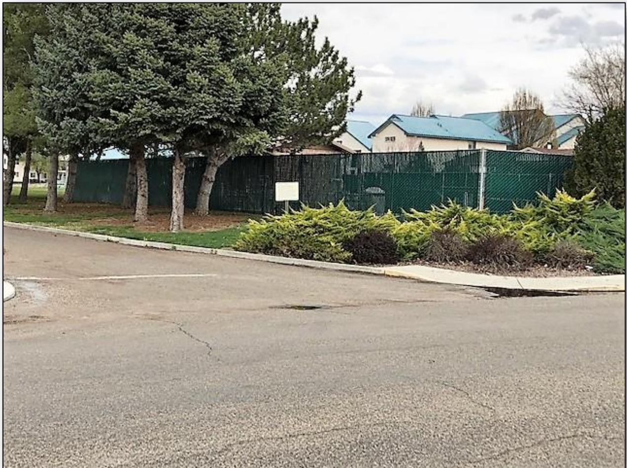
New chain link fence slats around 8 th Ave. lift station at Beck Kiwanis Park.
