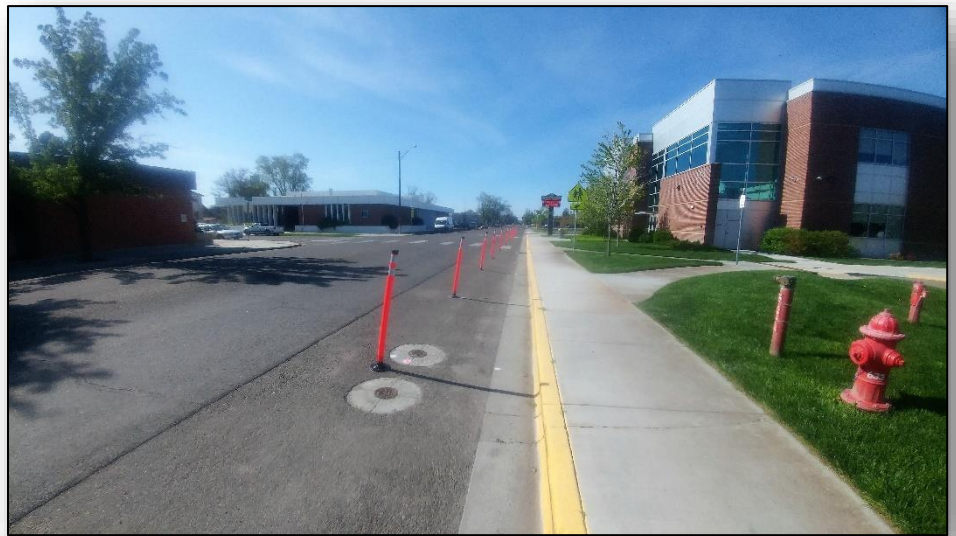
Newly installed delineator's at OMS school zone.
