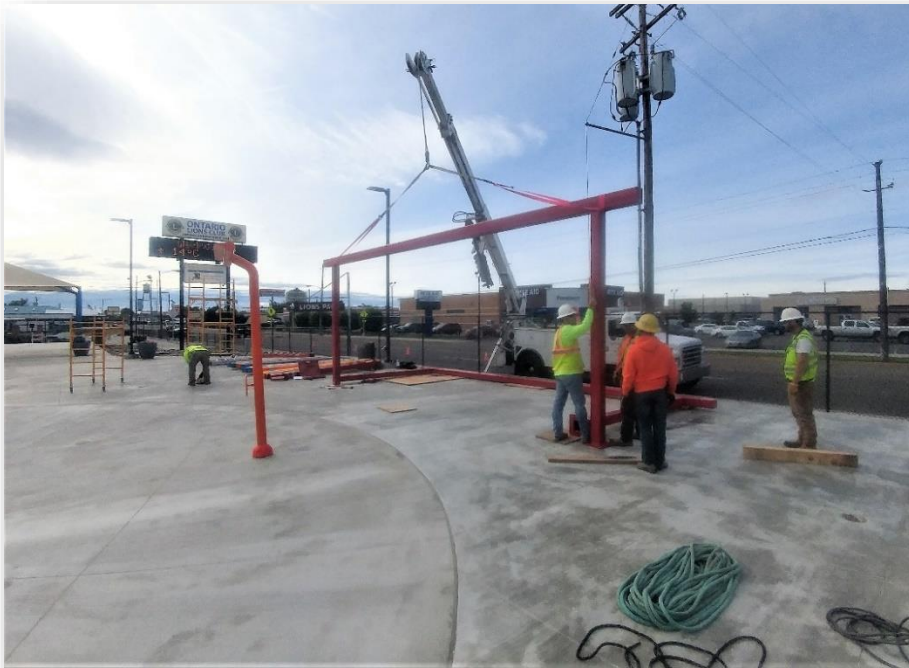
Both: Jacobs crew installing pergola at Splash Park.
