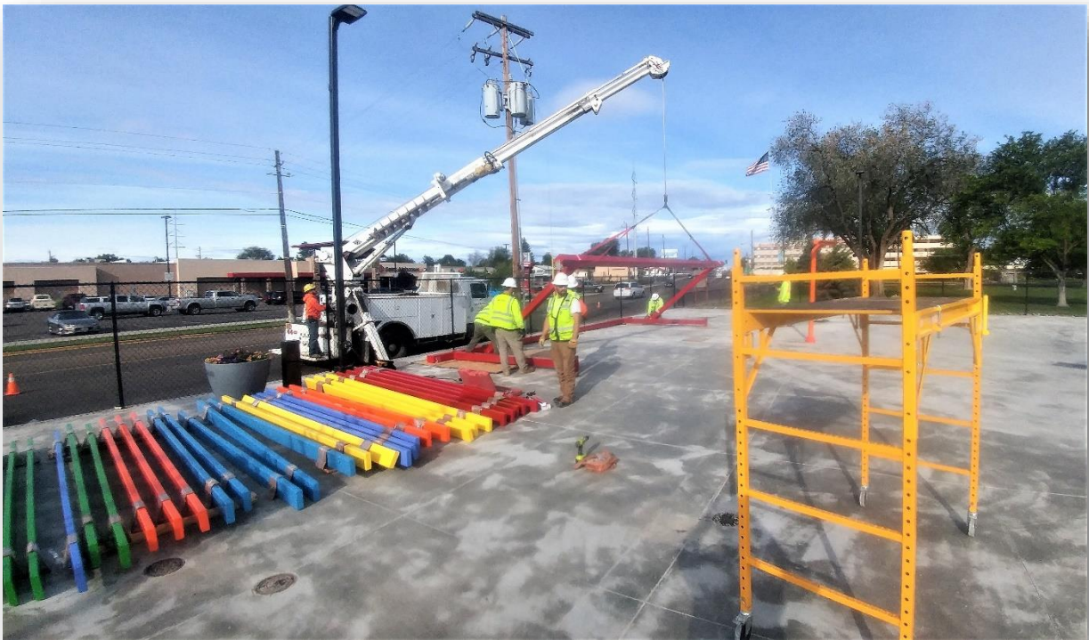
Jacobs crew installing pergola at Splash Park.
