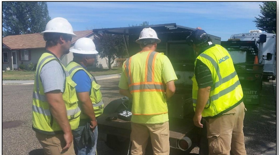
Bottom: Crews receiving training on new camera system.
