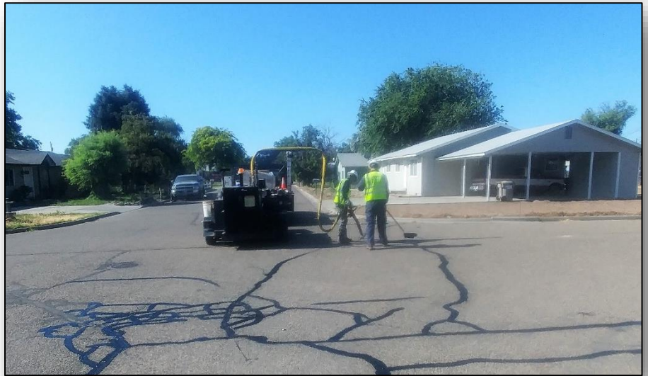
Top: Crews crack sealing in NW part of town.
