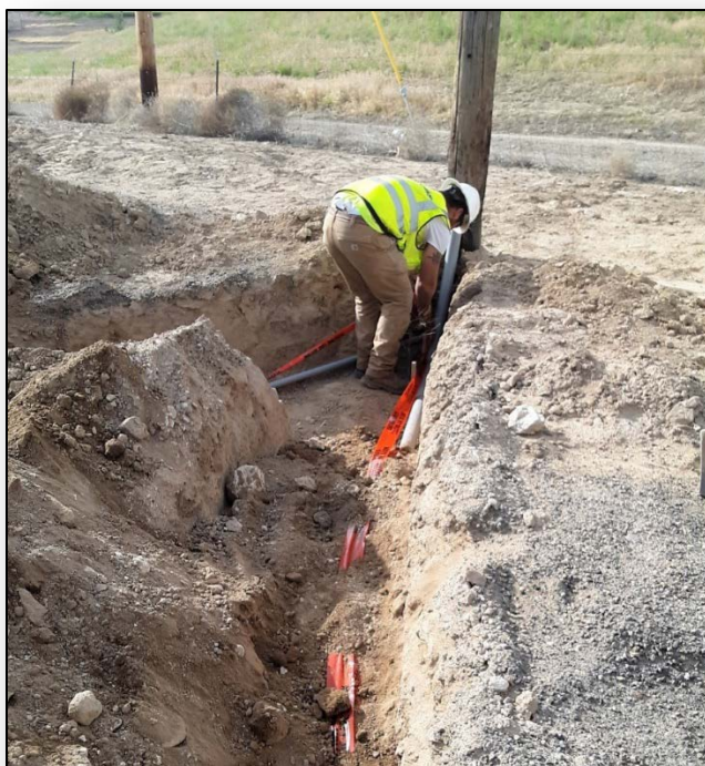
Bottom: Employee backfilling electrical trenches at Ontario Police Department gun range.
