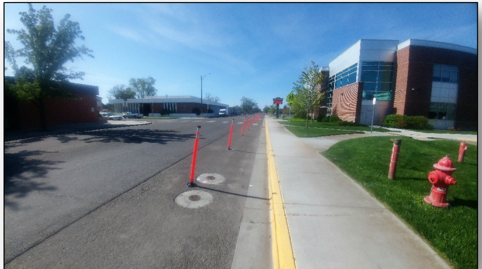
Newly installed delineator's at OMS school zone.
