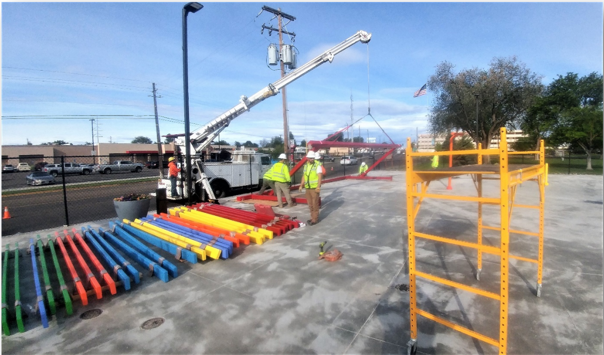
Jacobs crew installing pergola at Splash Park.
