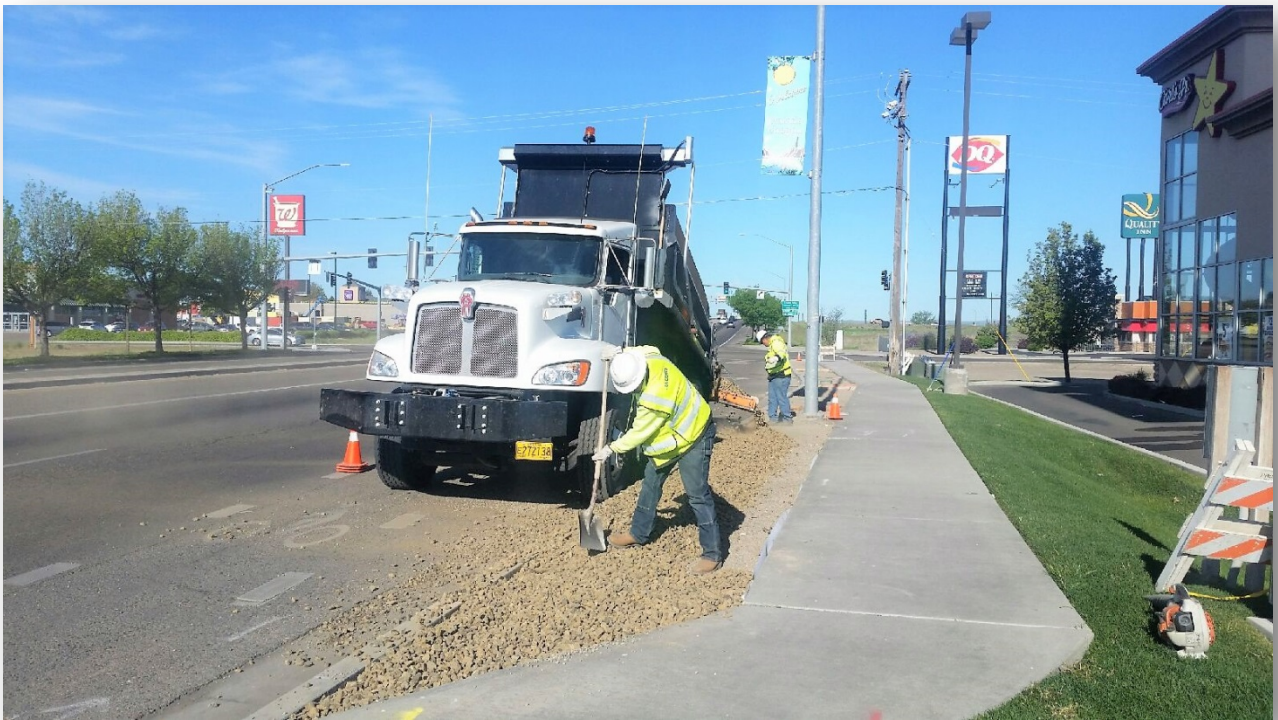
Jacobs crew installing new rock in planter strip on E. Idaho Ave.
