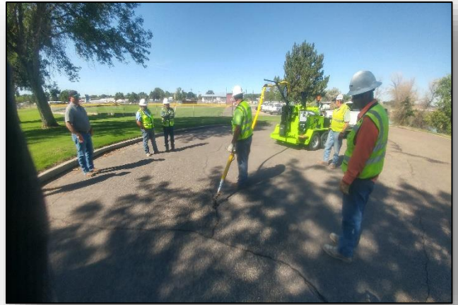
New Cimline crack seal training
