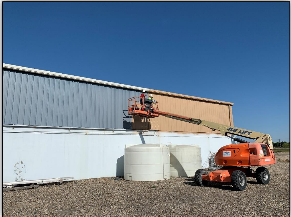
Jacobs staff painting the exterior of the old WTP
