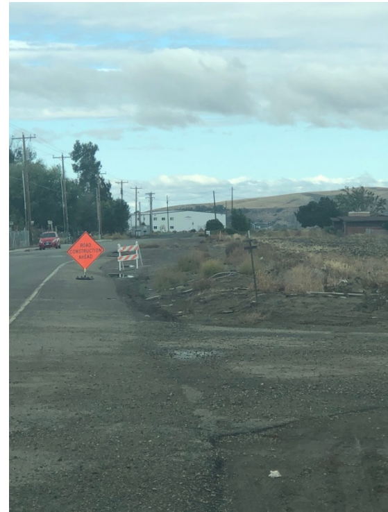
SW 4 th Ave – Parking Issues
