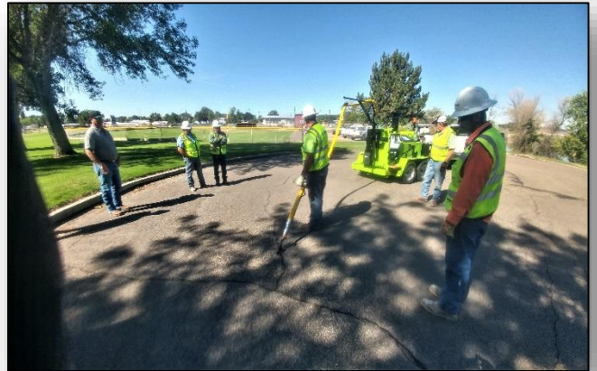
New Cimline crack seal training
