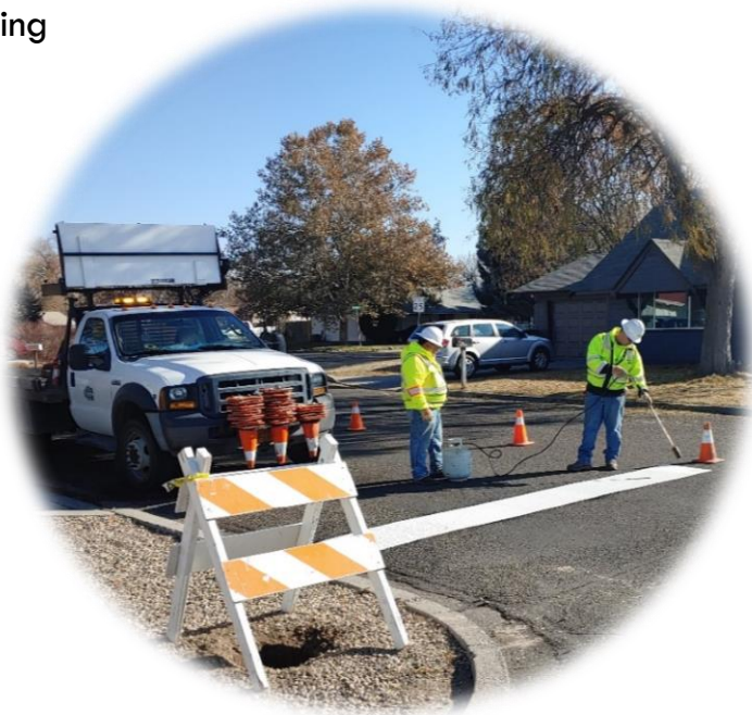
Right: Jacobs crew installing thermo plastic and stop sign.
