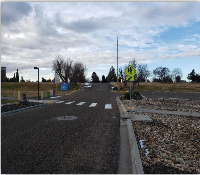
Above: Crosswalk signs on SW 11 th Ave at TVCC
