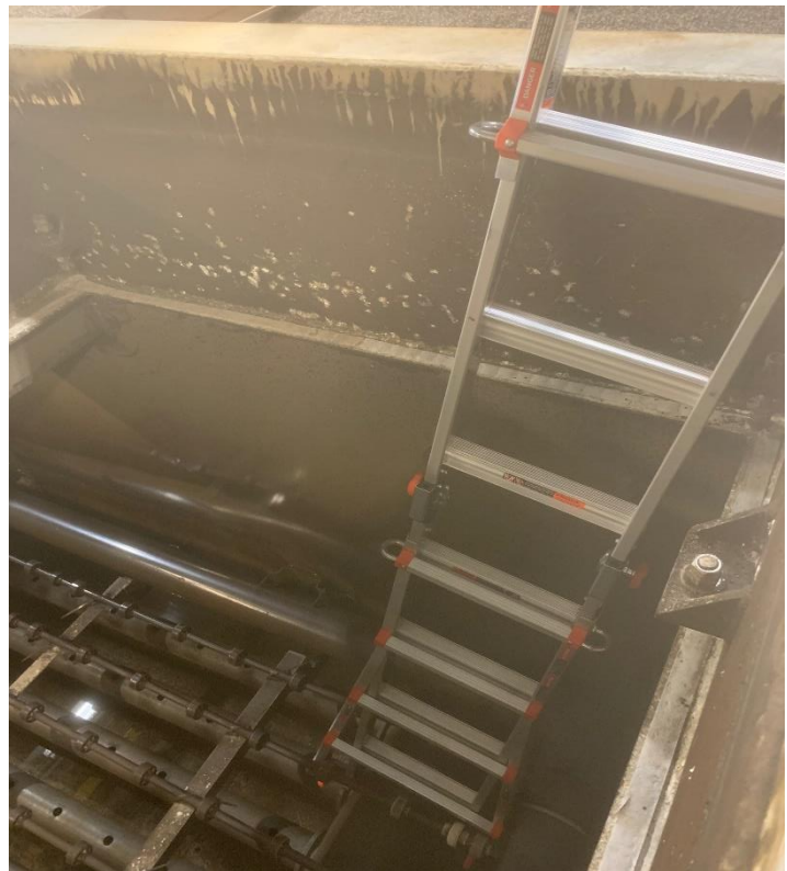
Below: Annual maintenance on WesTech clarifier #1
