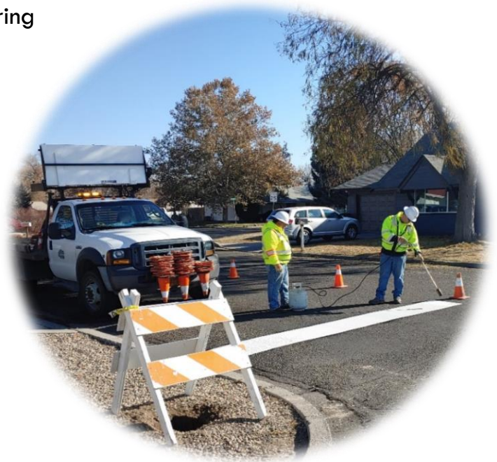
Right: Jacobs crew installing thermo plastic and a new stop sign.
