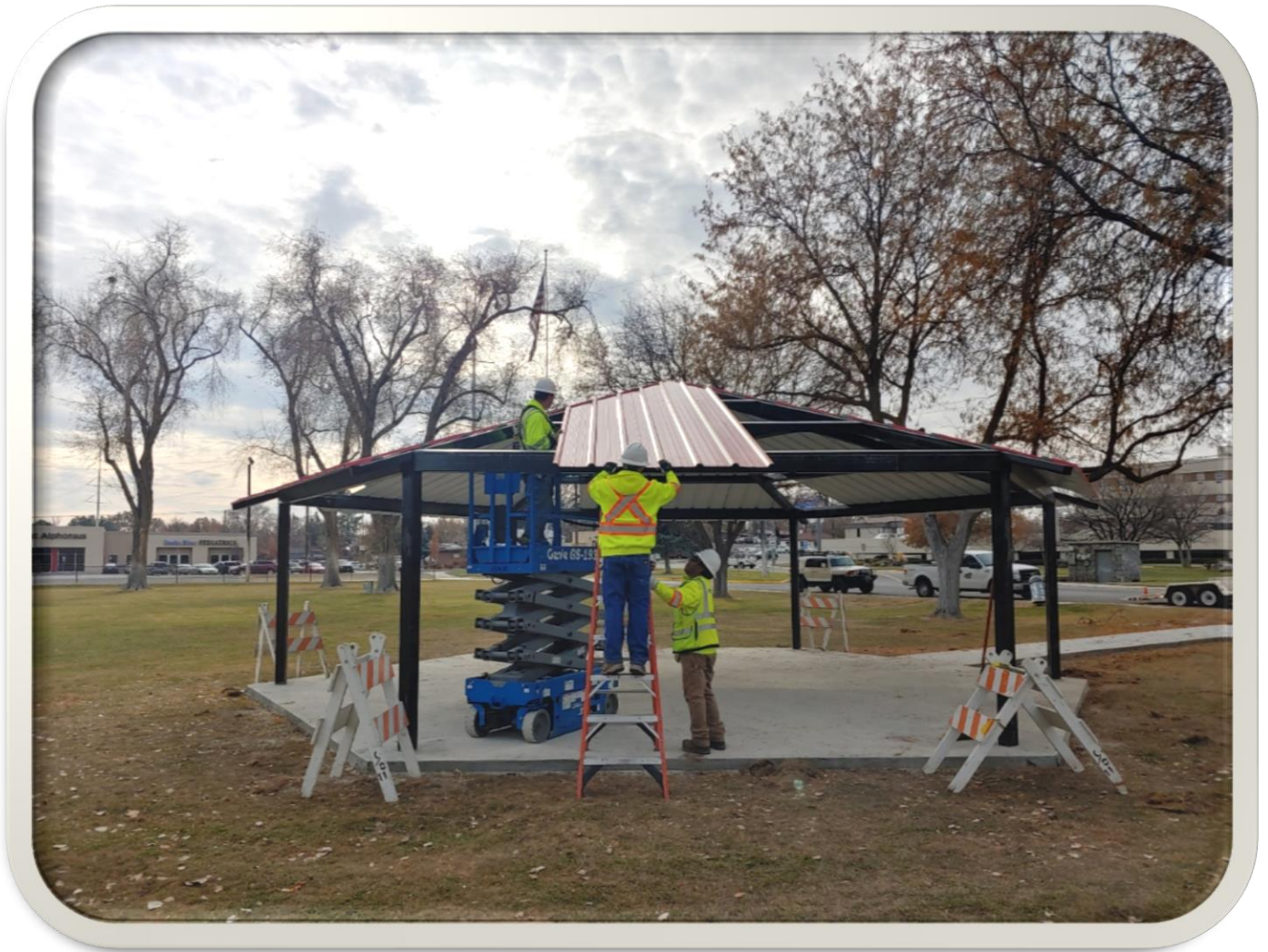
Above: Jacobs staff installing the roof on the shelter at Lions Park.
