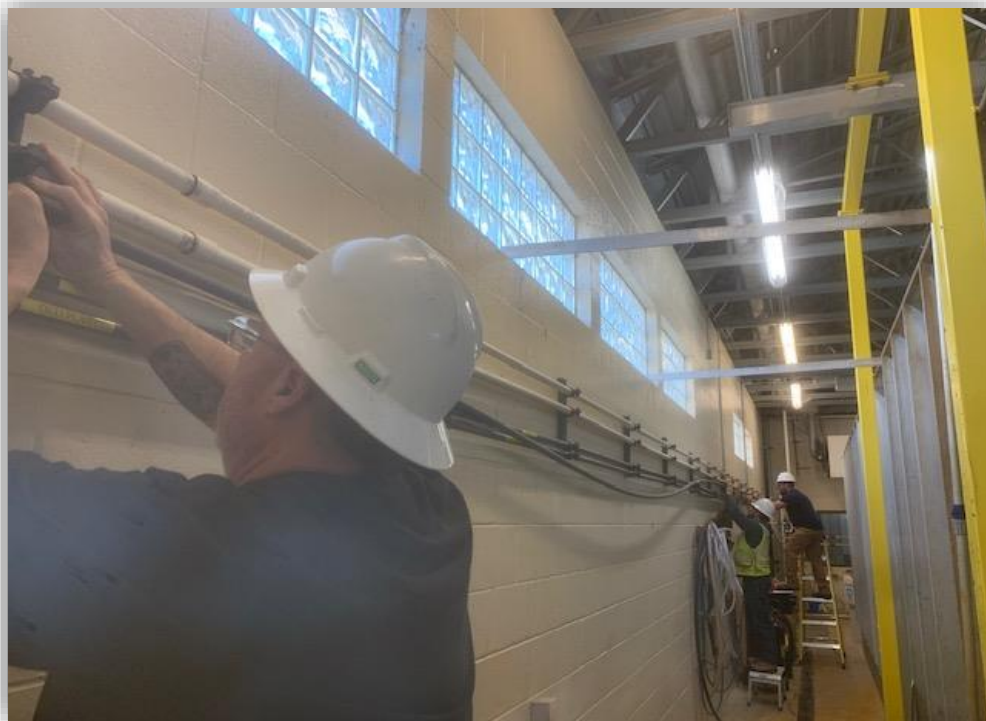
Jacobs staff installing new chemical lines at the Water treatment plant.
