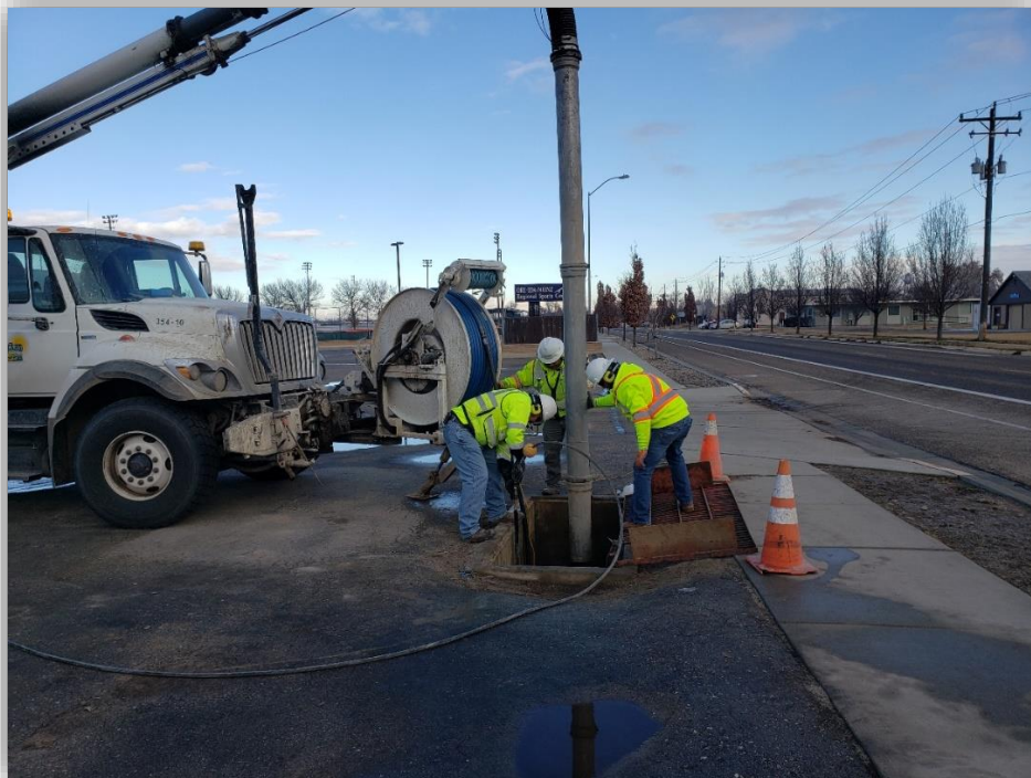
Above: Jacobs crew cleaning storm water line at TVCC with our jet rodding equipment.
