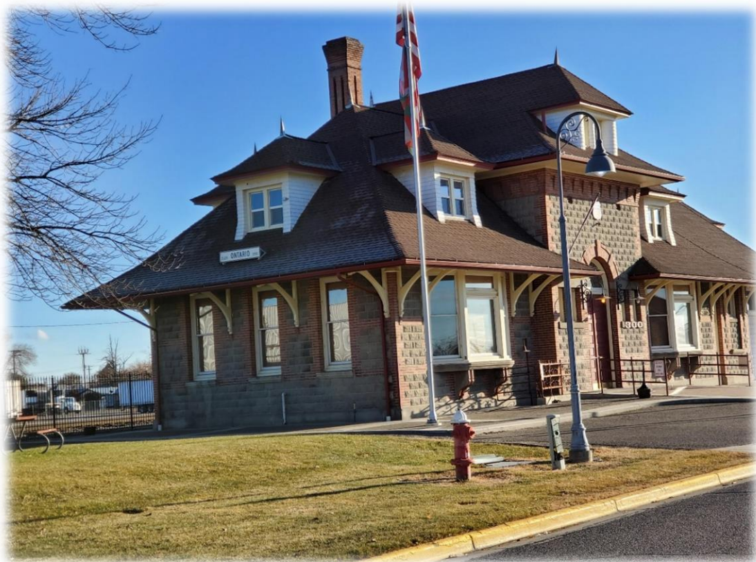
Ontario Train Depot
