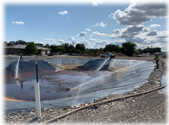
Right: Jacobs staff removing solids from wash water recovery basin #4 at the water treatment plant.
