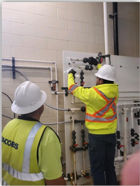
Above: Jacobs staff performing maintenance on KmnO 4 chemical feed line.
