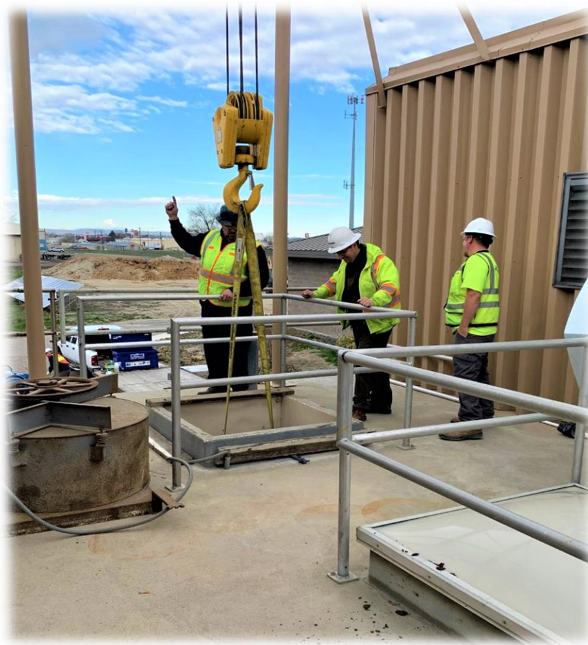
Jacobs Crew: Installing main distribution pump #4
