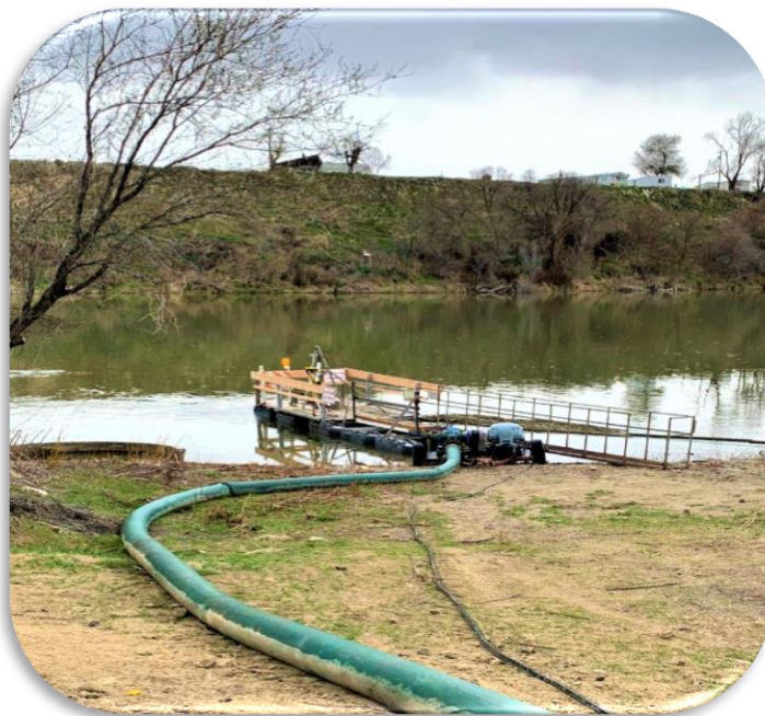
Auxiliary River pump after modifications to accommodate cleaning of the intake screen.
