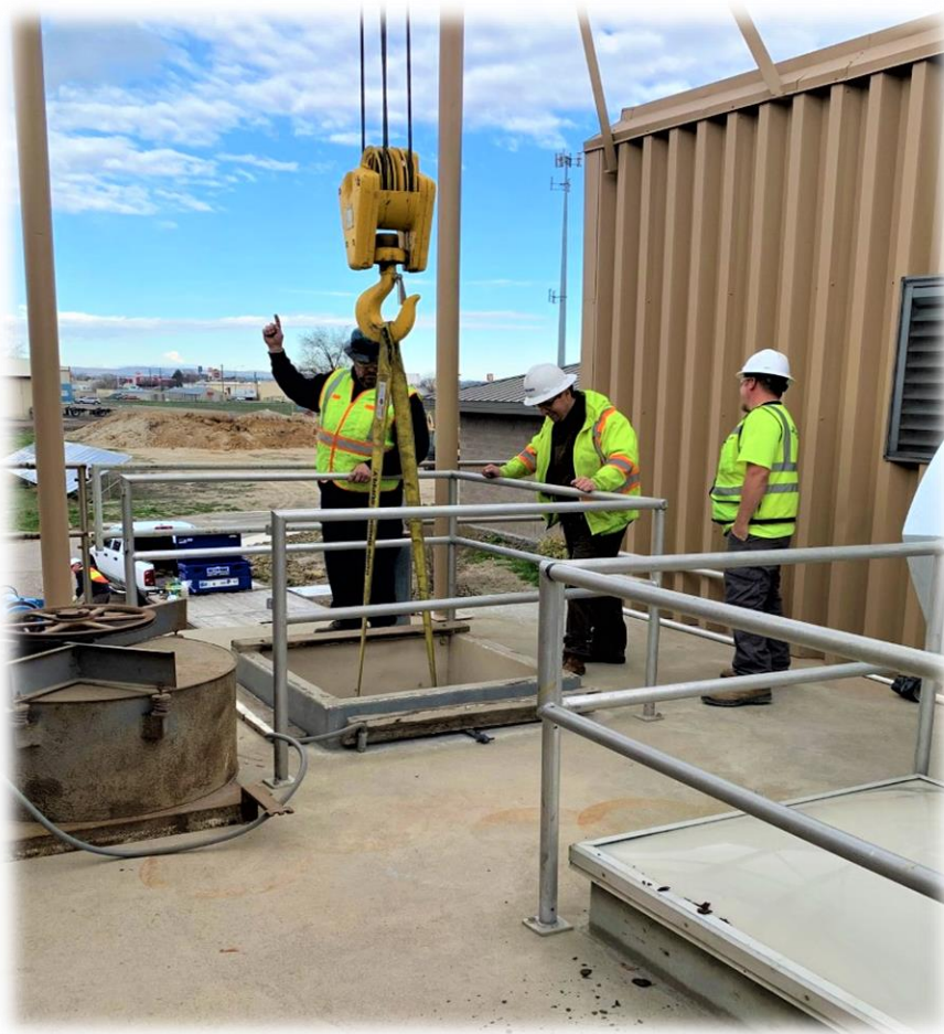
Jacobs Crew: Installing main distribution pump #4
