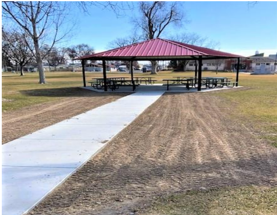
Dirt work done at Lions Park to prepare for planting grass.
