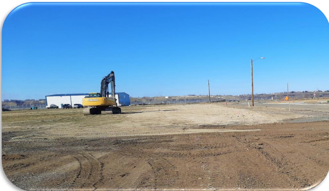
Work has begun on SW 33 rd Street Sewer Extension.
