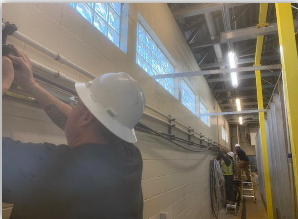
Jacobs staff installing new chemical lines
