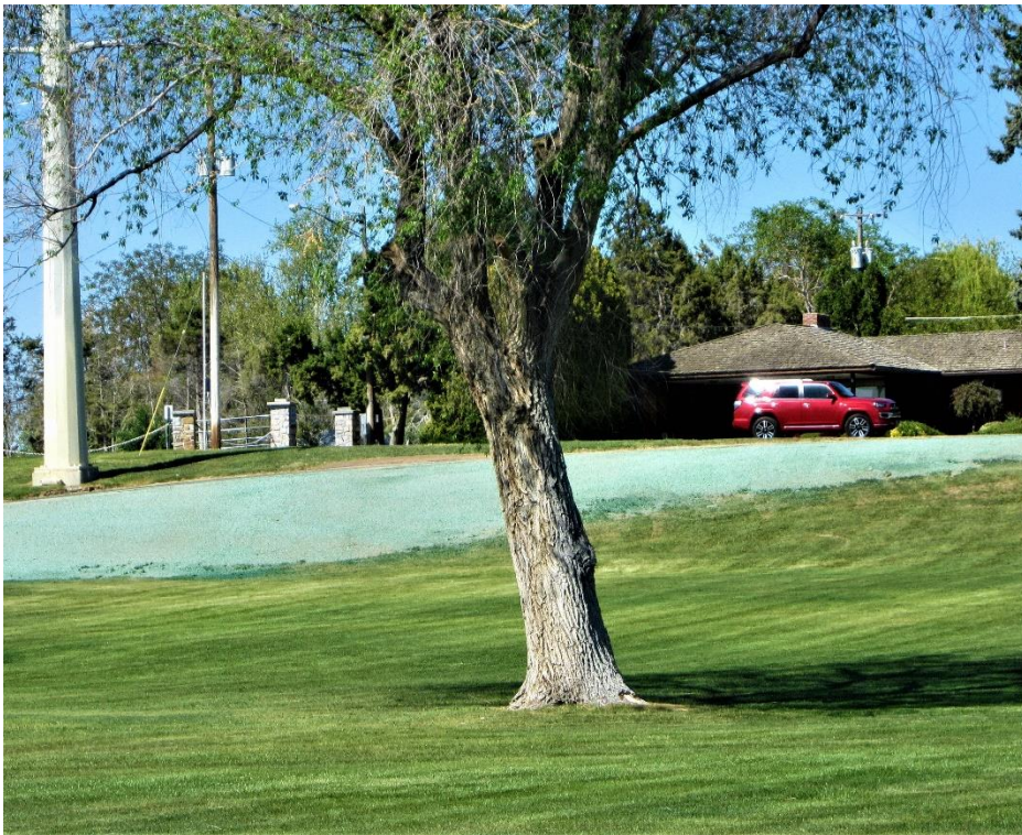
Hydro-seeding along the TV Connector Path.
