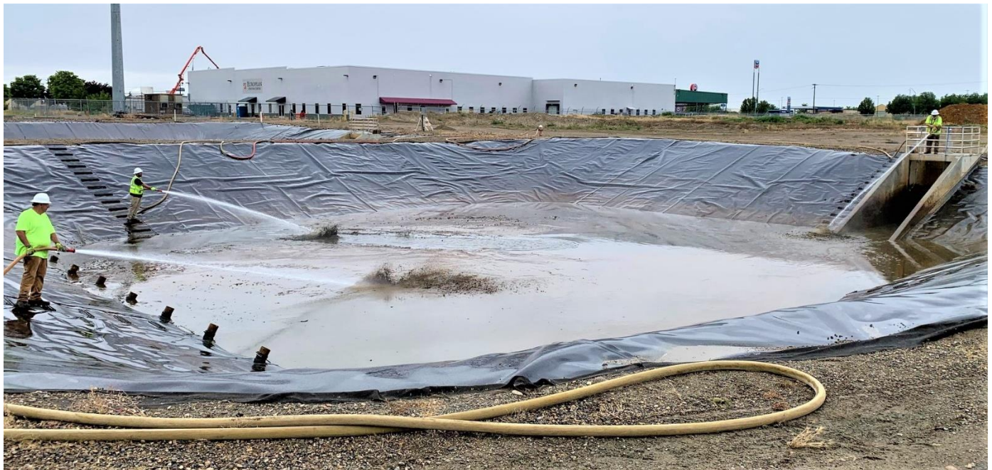
Jacobs Staff Members cleaning the wash water recovery basin #3 at the Water Treatment plant.
