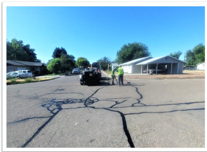
Jacobs Staff Members crack sealing roads.
