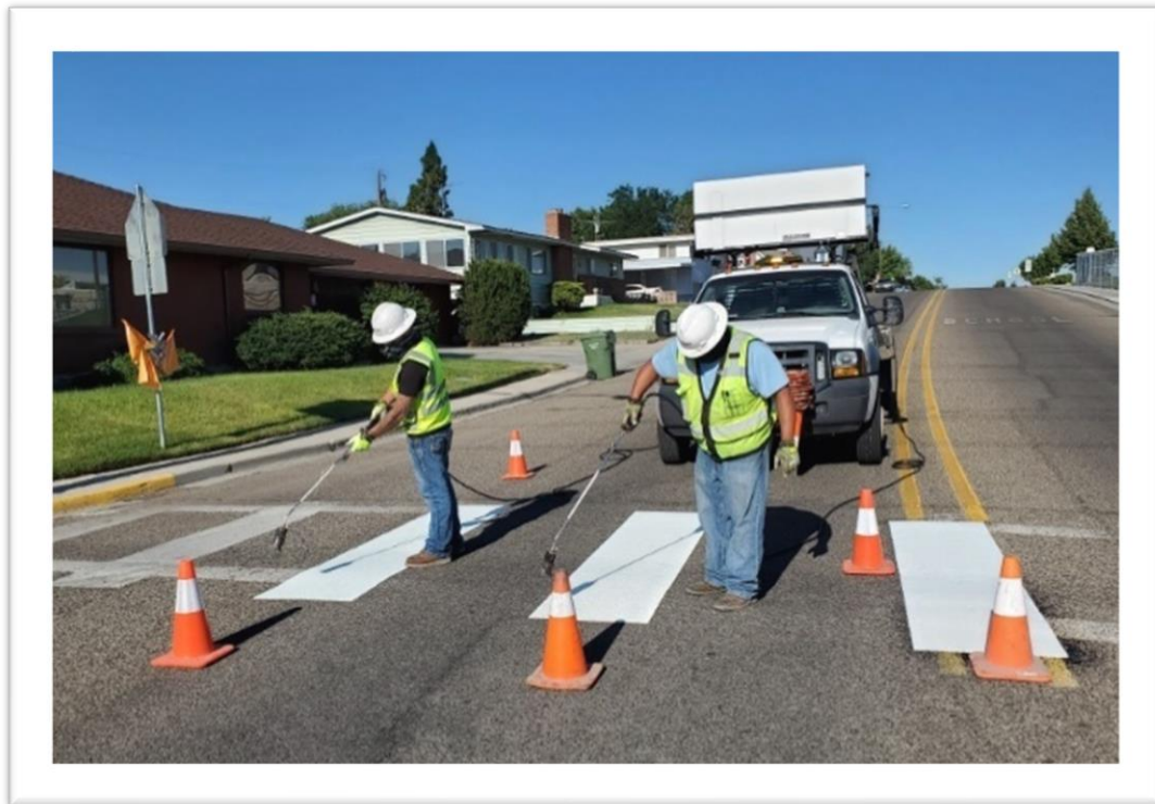
Jacobs Staff Members replacing the thermo plastic crosswalk.
