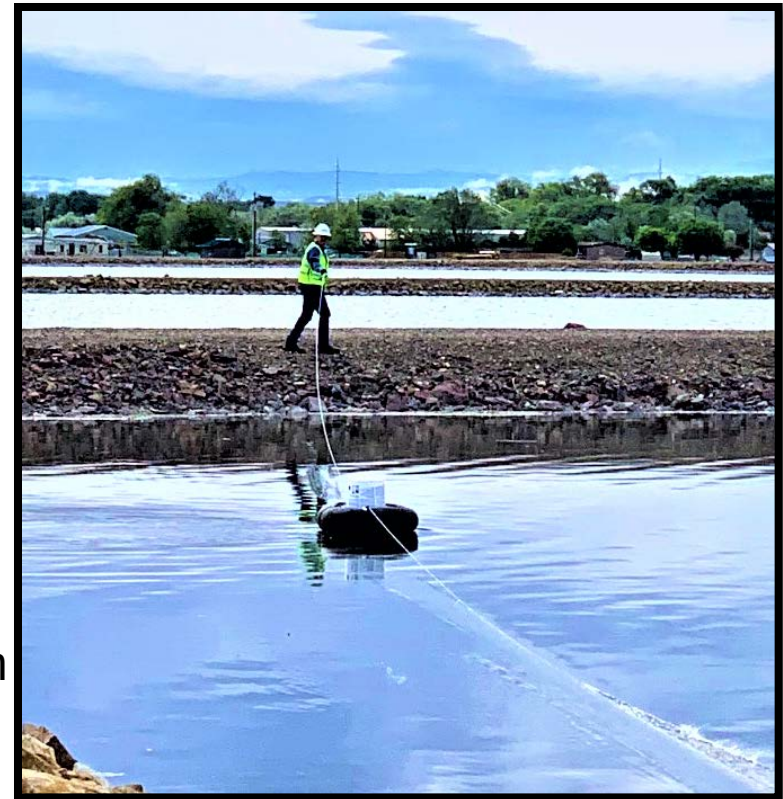
Left: Jacobs staff performing services to aerators in lagoon #1.
