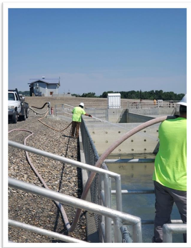
Jacobs staff members washing down the west chlorine contact chamber at the Wastewater Treatment Plant.
