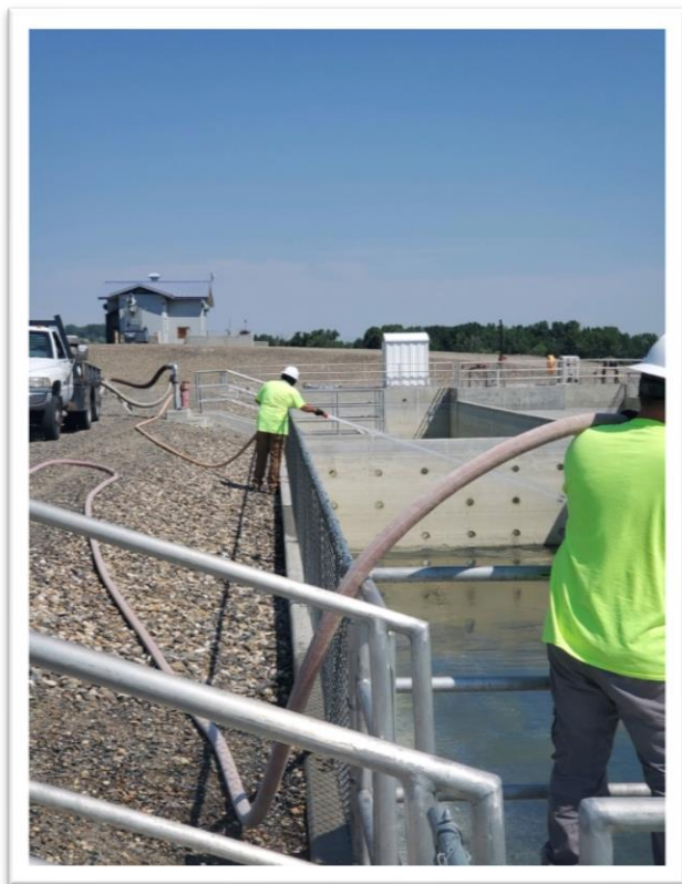
Jacobs Staff: Washing down the west chlorine contact chamber at the Wastewater Treatment Plant.
