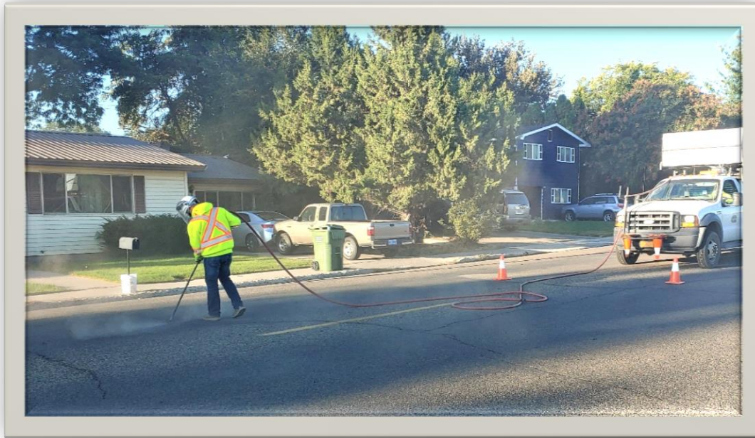
Jacobs Staff crack sealing the streets.
