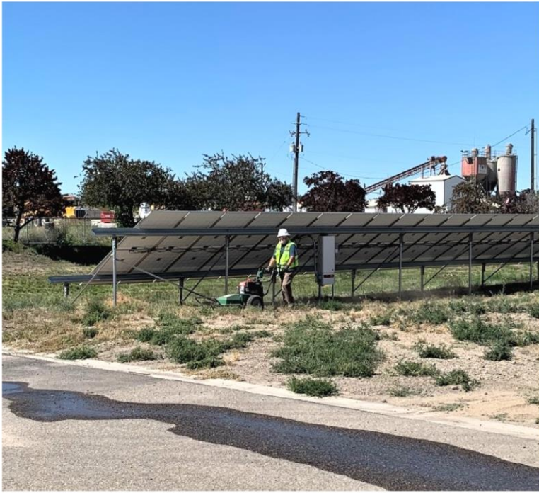
Upper Left: Jacobs Staff performing weed maintenance at Water Plant.
