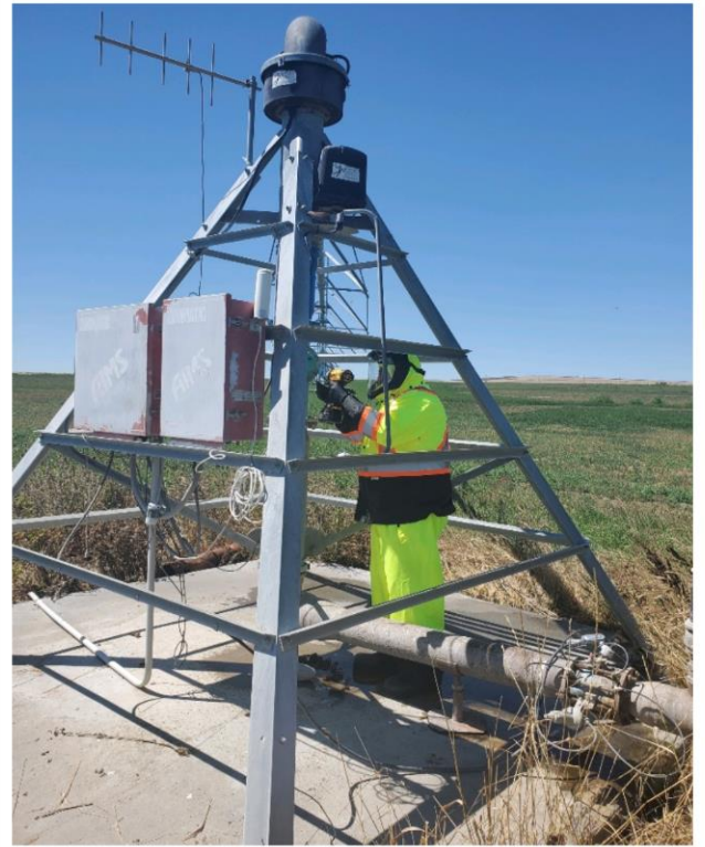
Upper Right: Jacobs Staff replacing flow meter on Skyline pivot #1.
