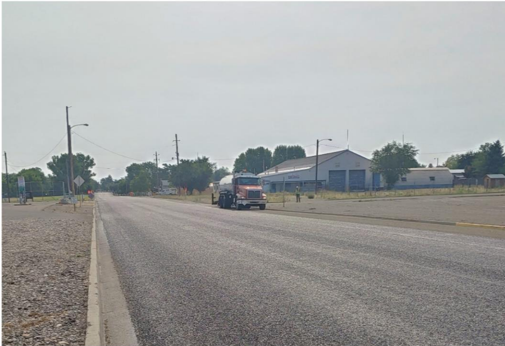
Top: Fog sealing the road.
