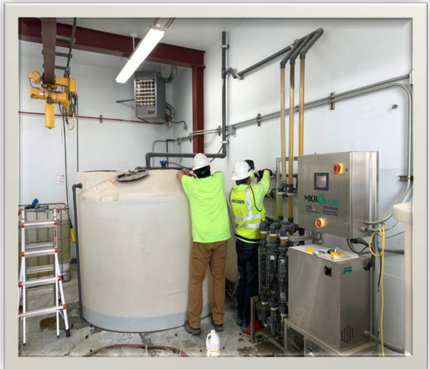
Right: Jim Raynor and Kenny Nelson performing maintenance on the chlorine storage vessel at the Wastewater Treatment Plant.
