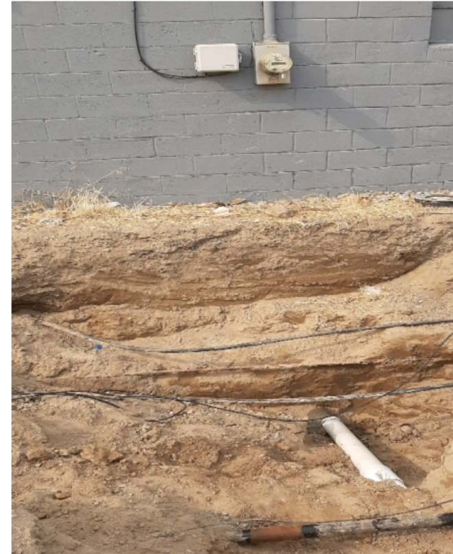
Sewer service installation inspection
