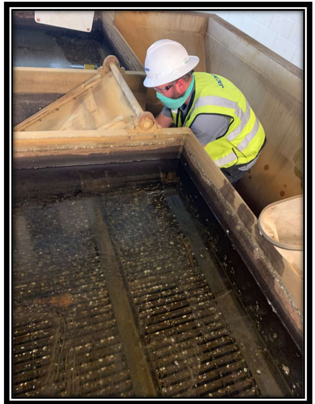
Below: Robert Crites Performing an Inspection of the WesTech Water Treatment Train #2 Wastegate.
