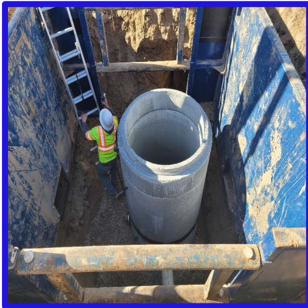
New sewer manhole that a contractor is installing along Arcata Way and SW 18th St at Sunset Estates Phase 2.
