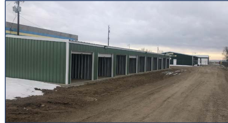
Ontario Mini Storage 2252 SW 4 th Ave Under Construction
