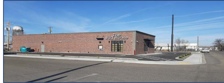
The Bud House 215 NE 2 nd Street Under Construction
