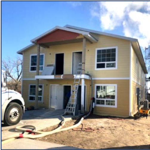
754 River Street Fourplex Under Construction
