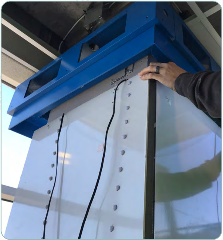
LED Enclosure Installation
