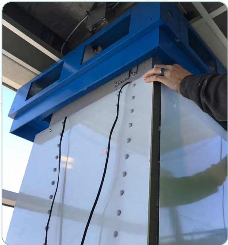
LED Enclosure Installation
