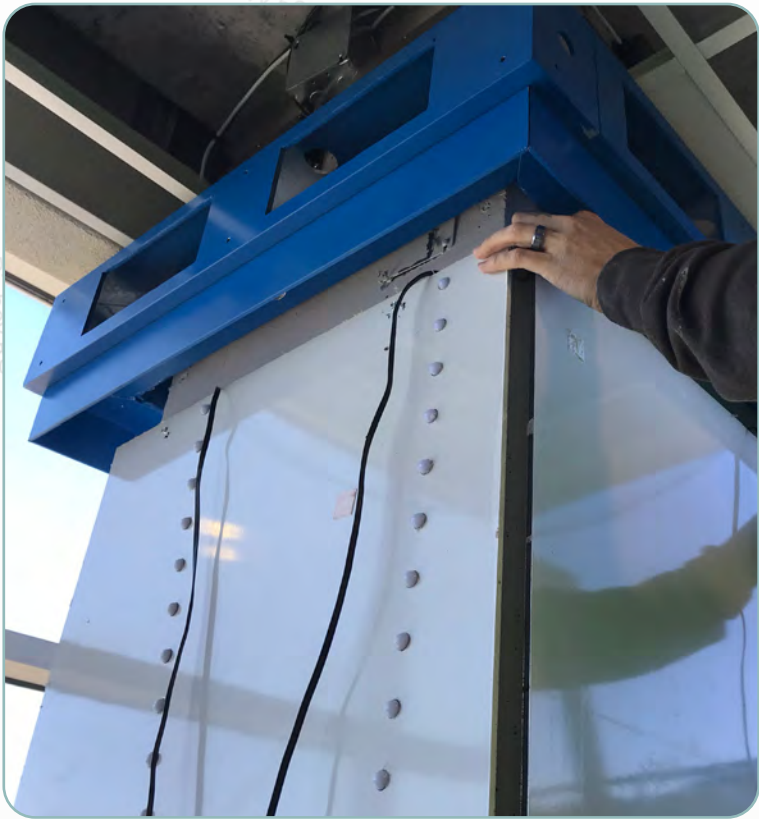
LED Enclosure Installation
