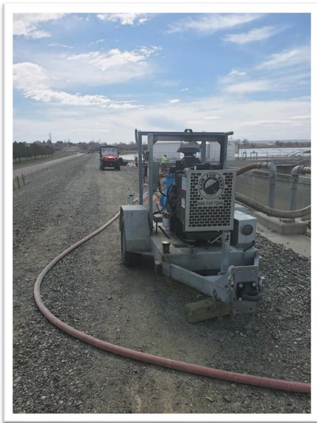
Cleaning east chlorine contact chamber at the Wastewater Treatment Plant.
