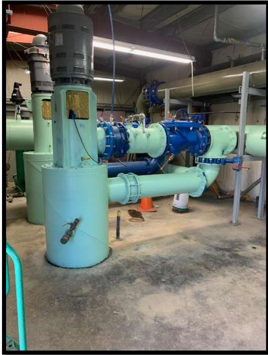
Above: Newly Painted River Pump Below: Filter #2 effluent Valve Removed for Service
