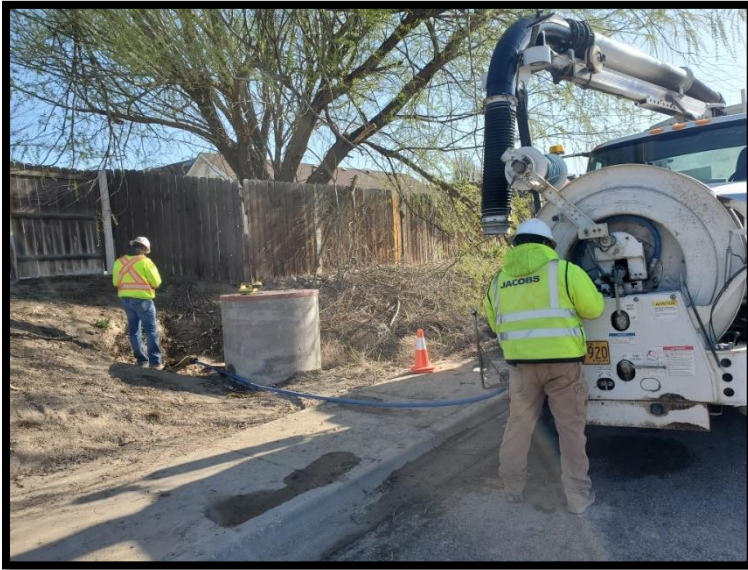
Cleaning Storm Hot Spots prior to Irrigation.
