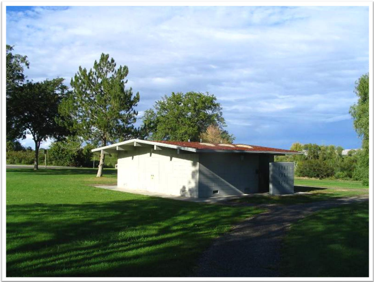
Ontario State Recreation site Restroom Building
