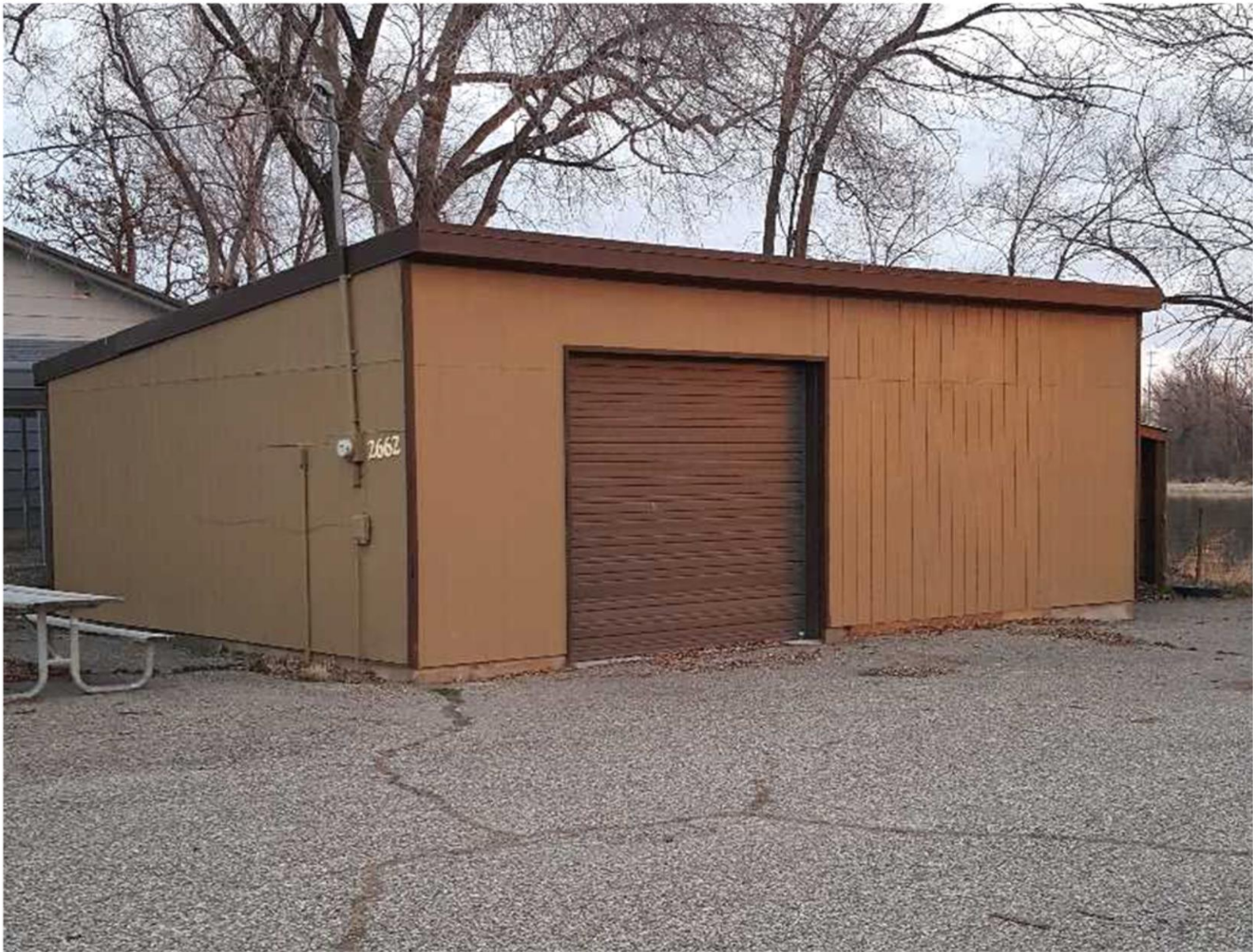
Maintenance Shop building
