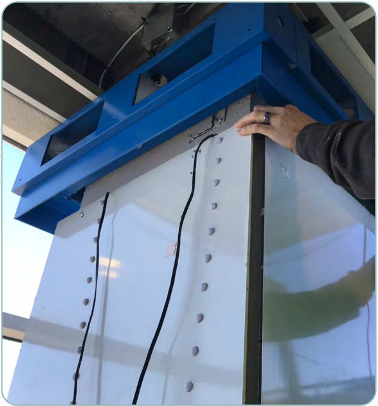
LED Enclosure Installation
