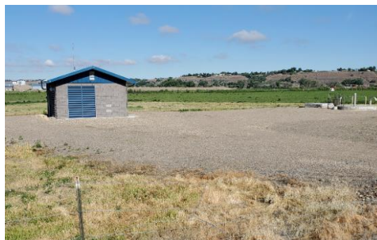
NW Regional Lift
