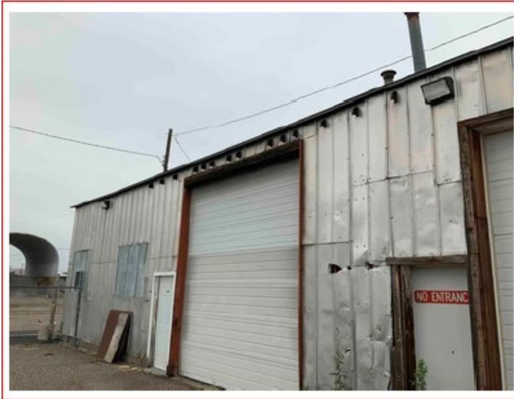
Figure 8. Old Public Works Bilding
