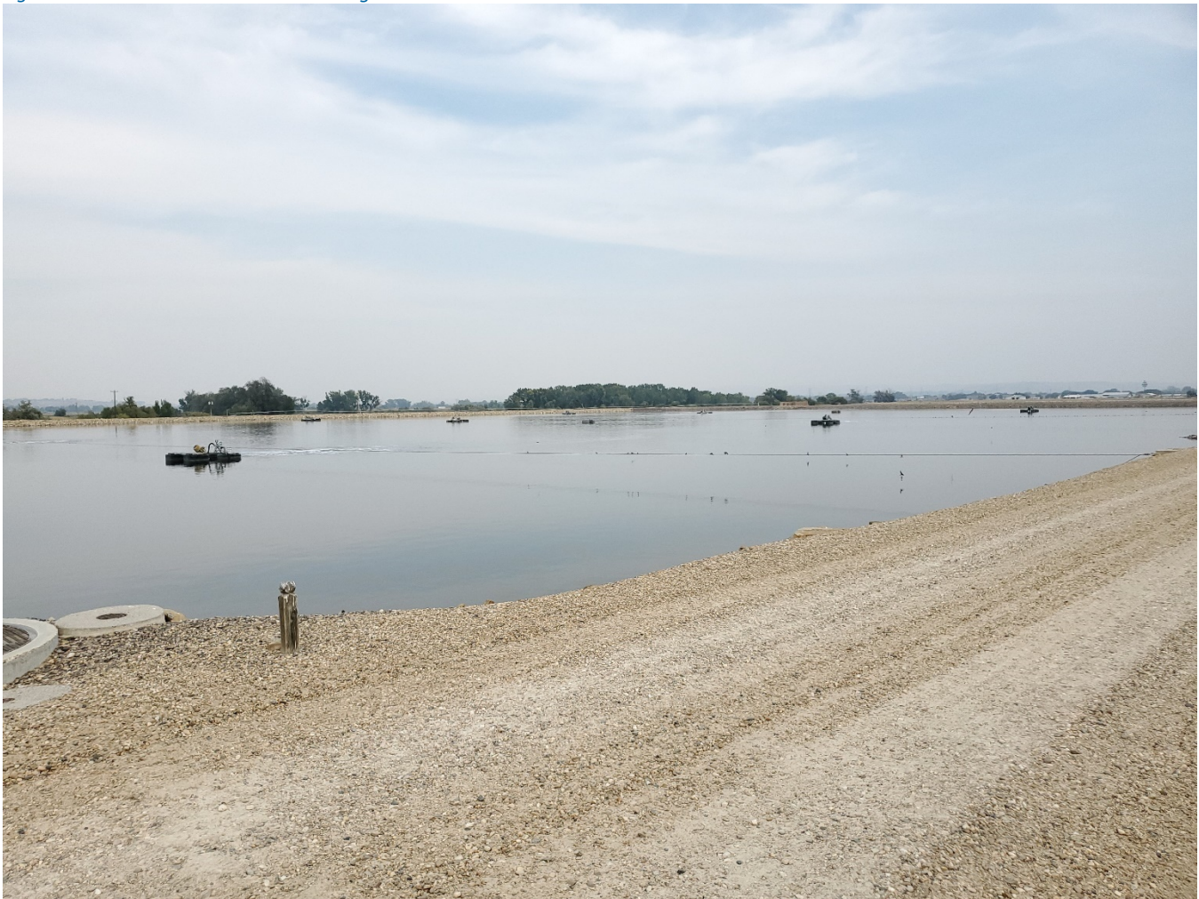
Figure 9. Wastewater Treatment Plant Lagoon #1
