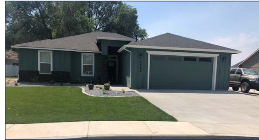
BK Construction Completed
