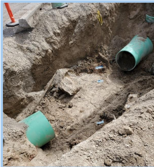
27" Storm line being relocated for new development
