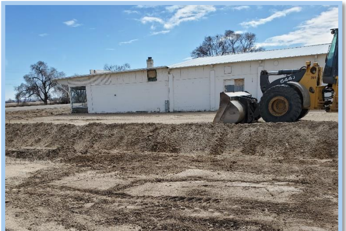
Storm Swale for new street section of Airport Way
