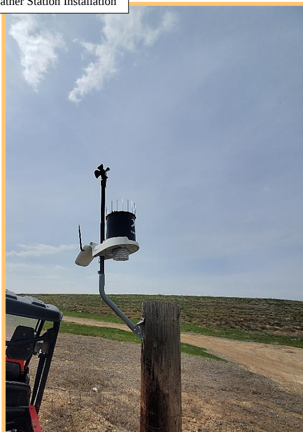
Weather Station Installation
