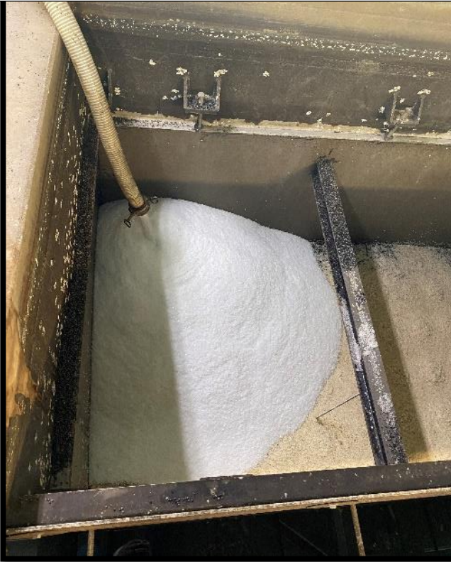
Installed new buoyant media in WesTech #2 Clarifier
