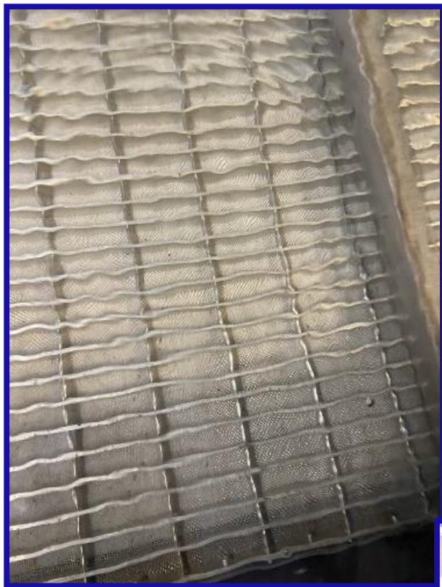
Installed new buoyant media retention screens
