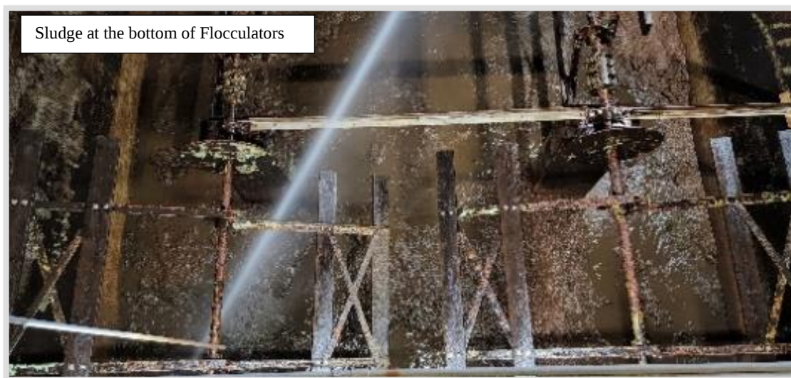
Prepping for work on Flocculator drive chain
