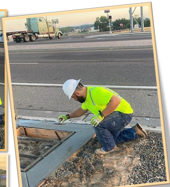
Pouring tree wells on E. Idaho Ave.
