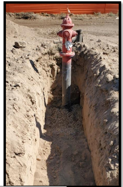
Install of Hydrants at Terranova Park
