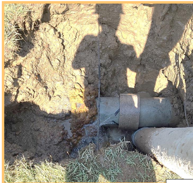
Water line Leak
